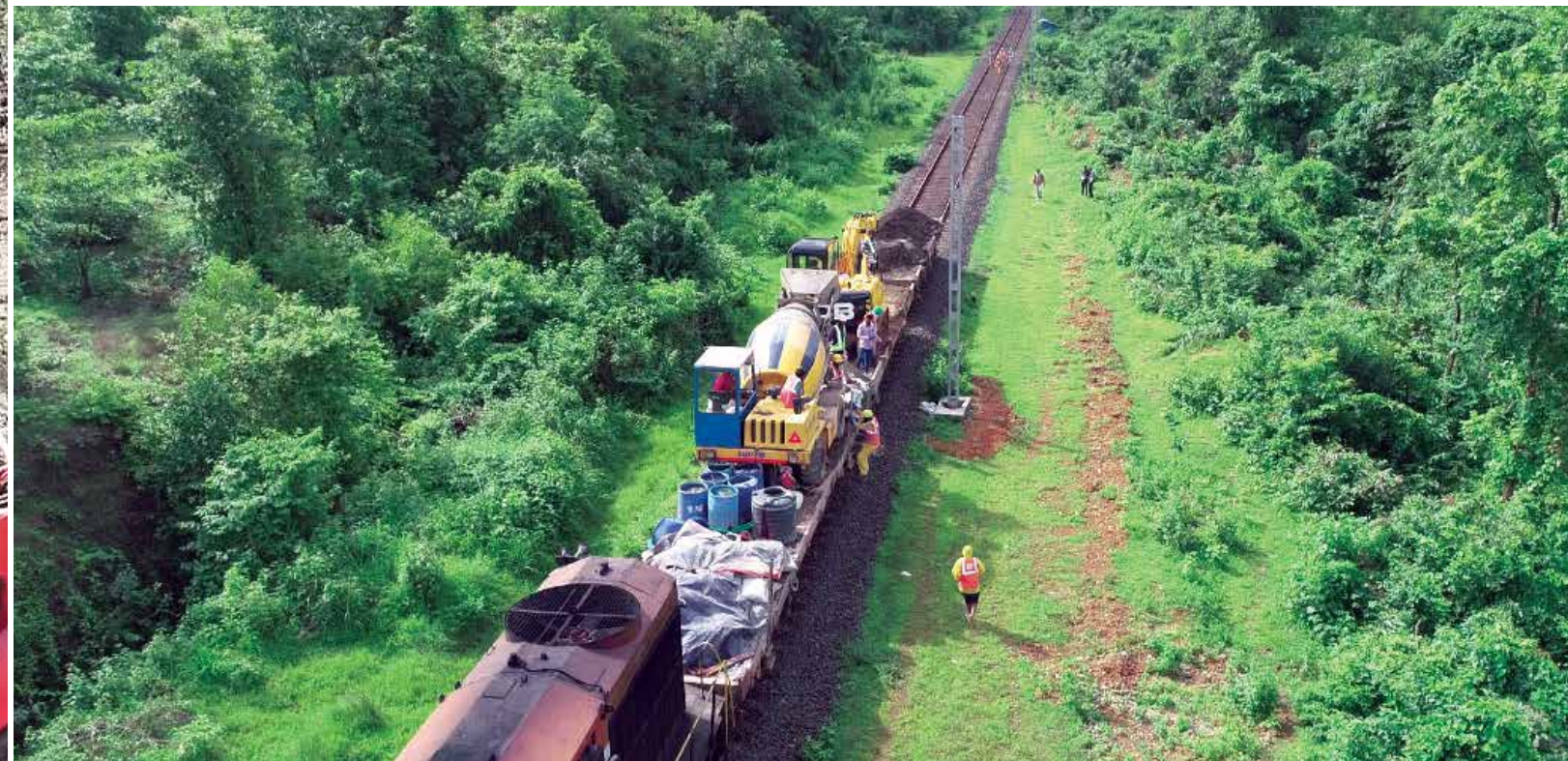
OHE foundation and mast erection at the Roha - Verna section
