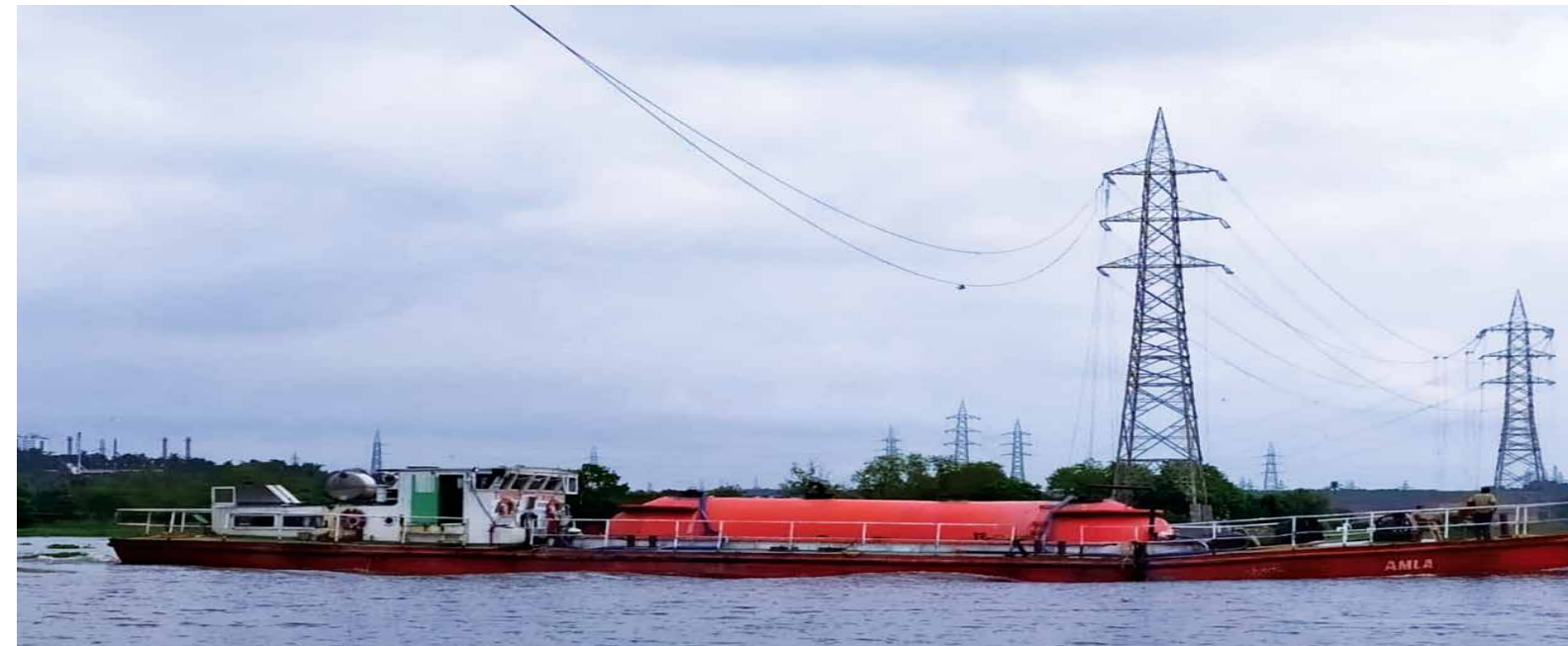
Stringing across a river at the 220/110 kV Kochi Transmission Line Project
