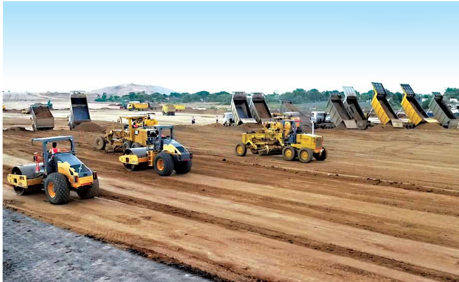
Soil embankment works in full swing at the Mallannasagar Reservoir Project
