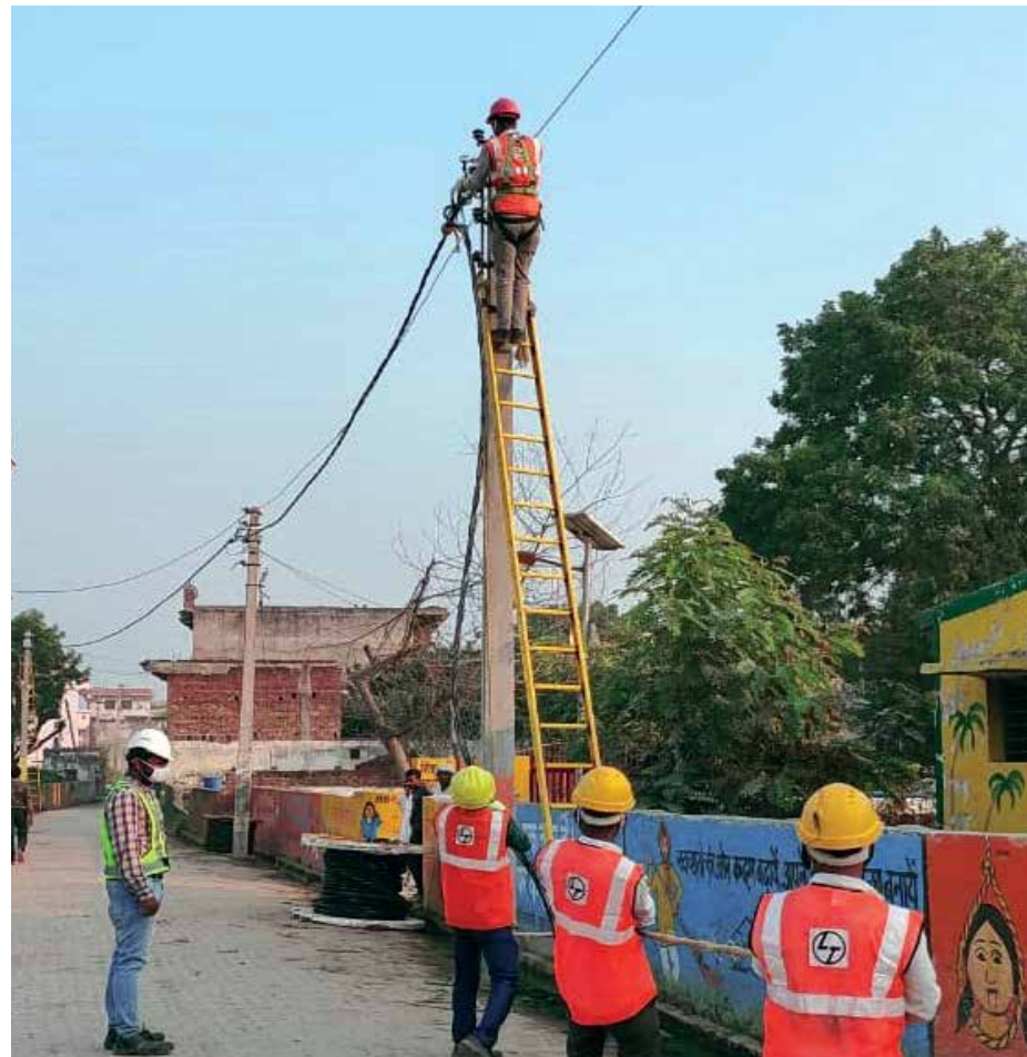
AB cable laying at Saubhagya Project
