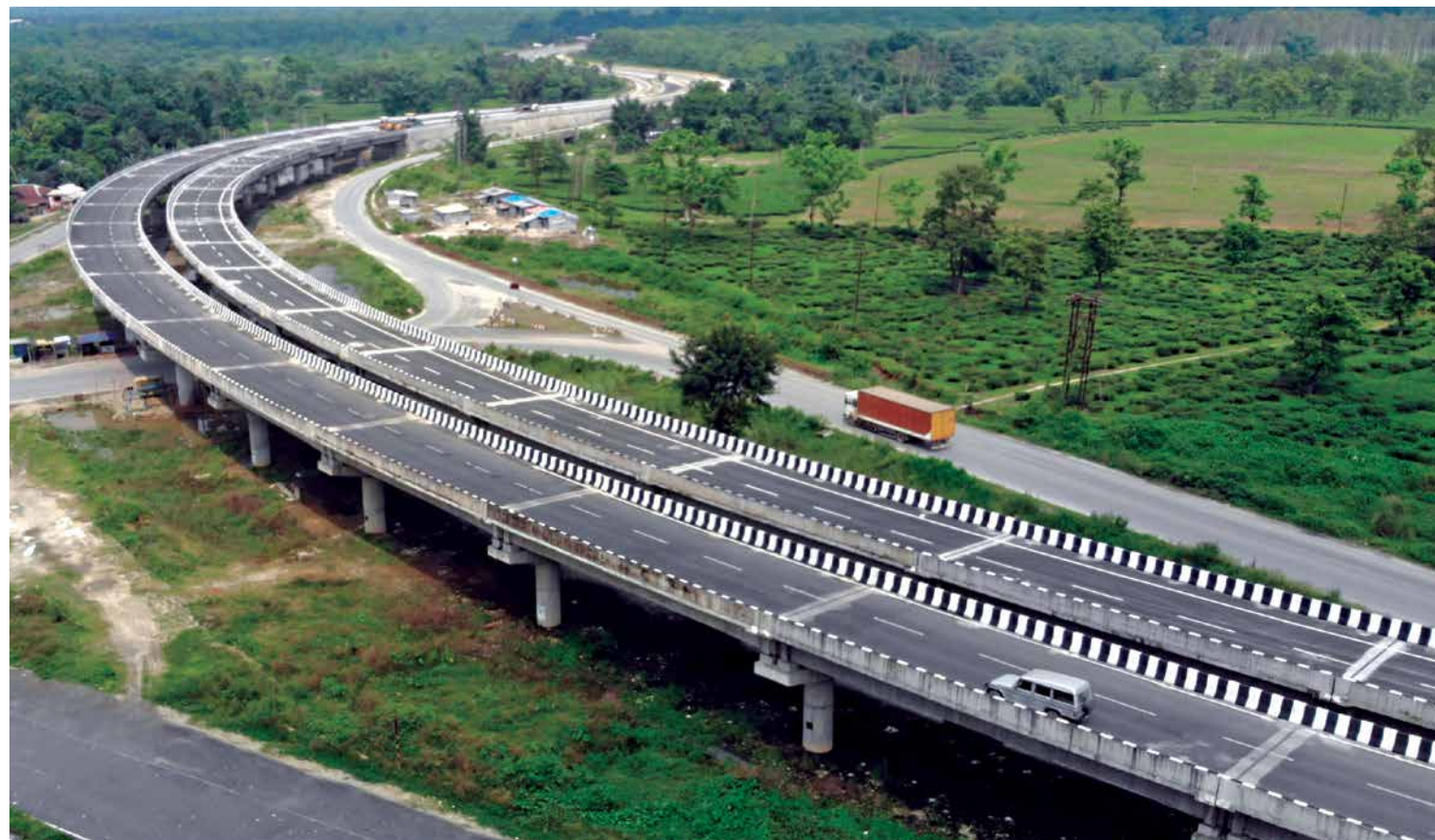
Flyover at Ghoshpukur
