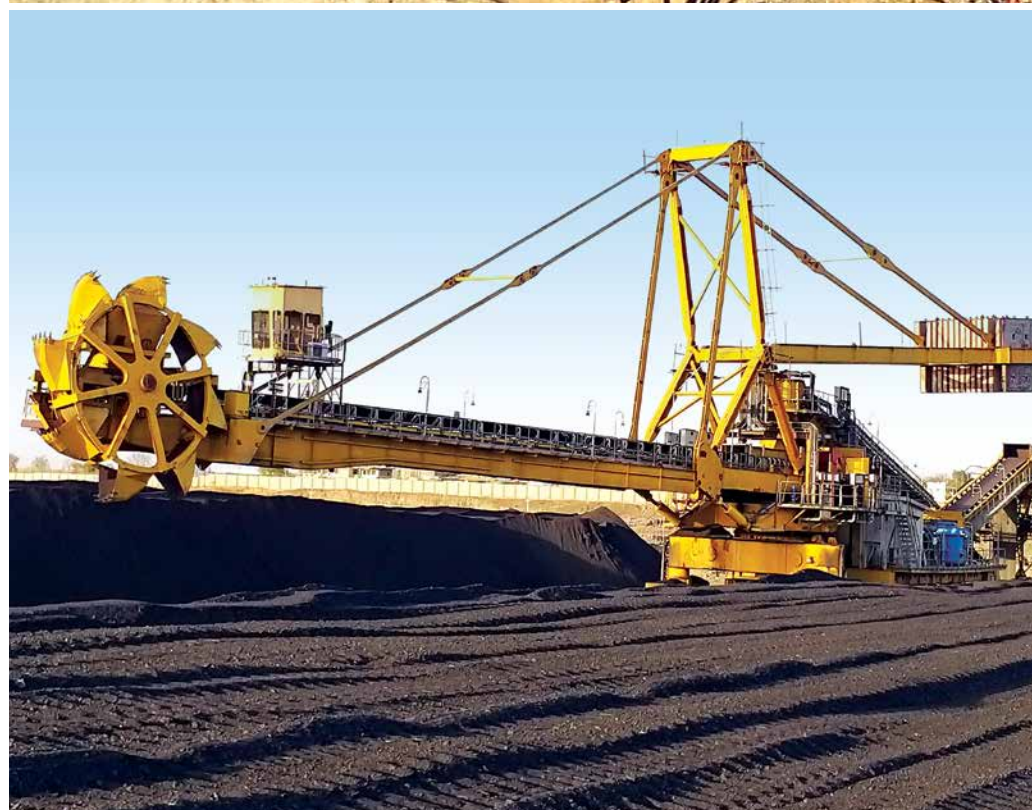
A stacker reclaimer at work at the CHP package, NTPC Khargone
