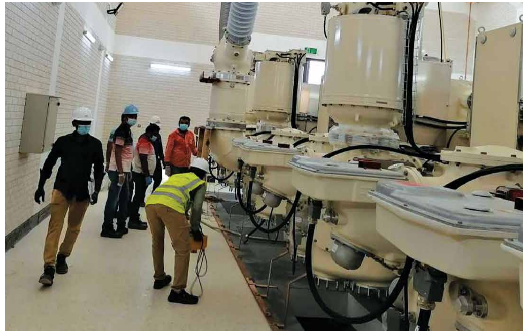
132 kV GIS HV testing at PAHW, Kuwait
