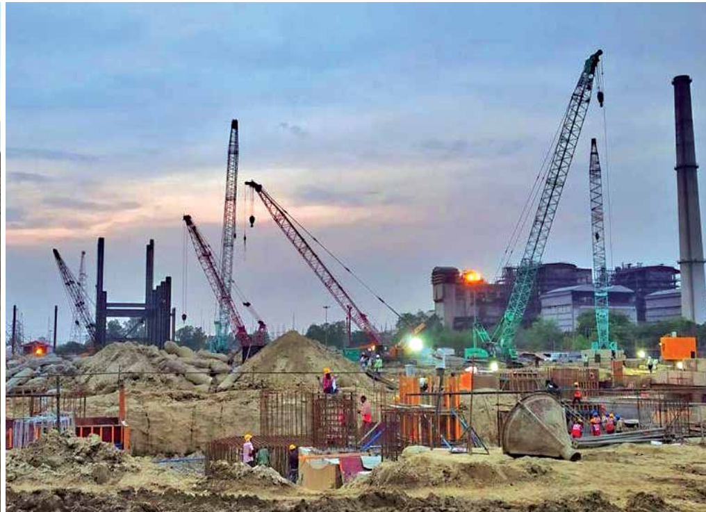
Piling work in progress at Panki
