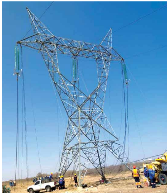
Stringing works across the 400 kV Morepule B–Orapa–Mawana Project, Botswana
