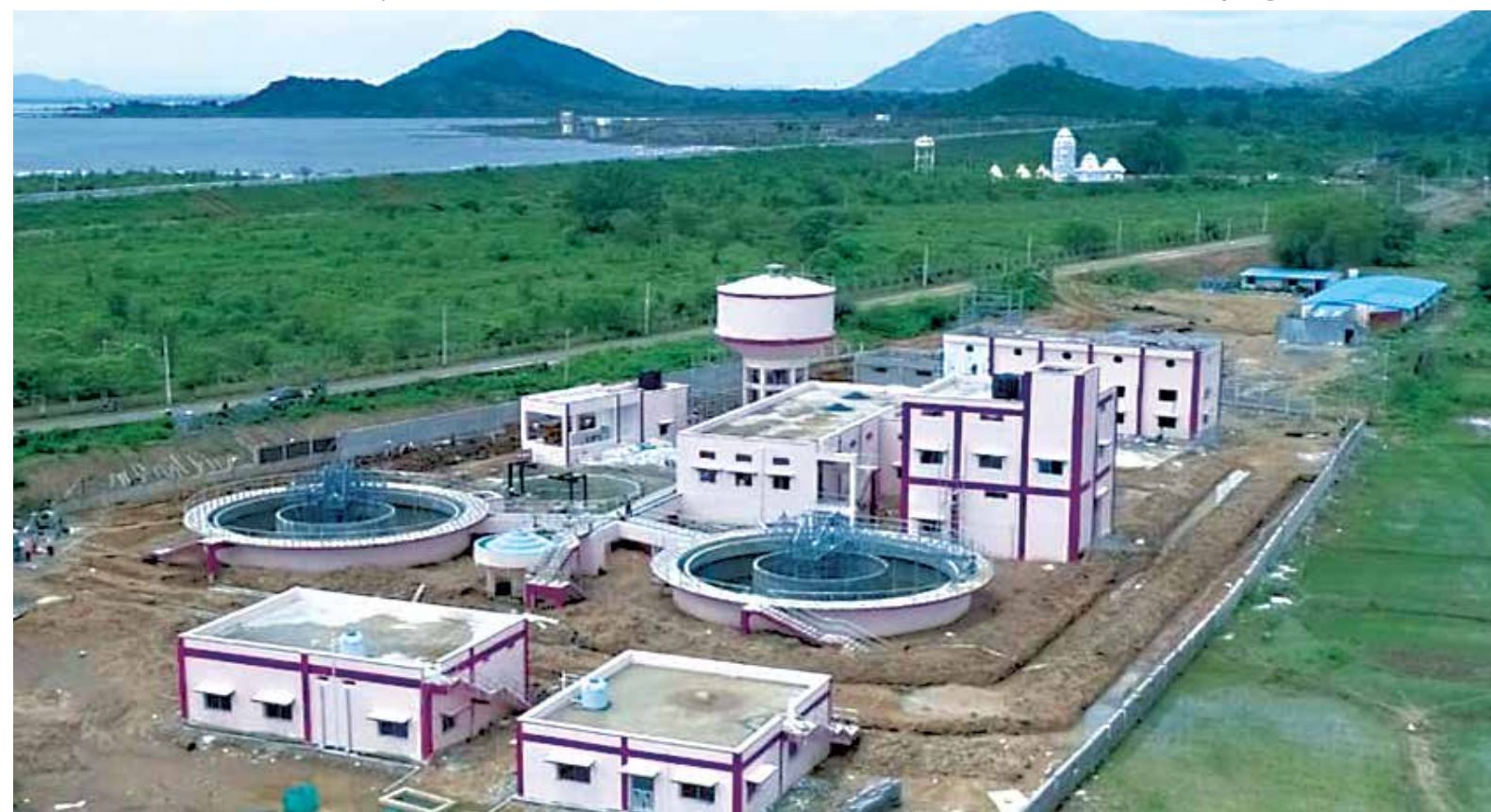
Nuapada WSS Plant on course for a scheduled completion
