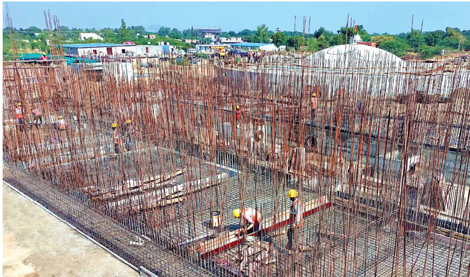
Construction of filter house at Jawai Cluster IV Project
