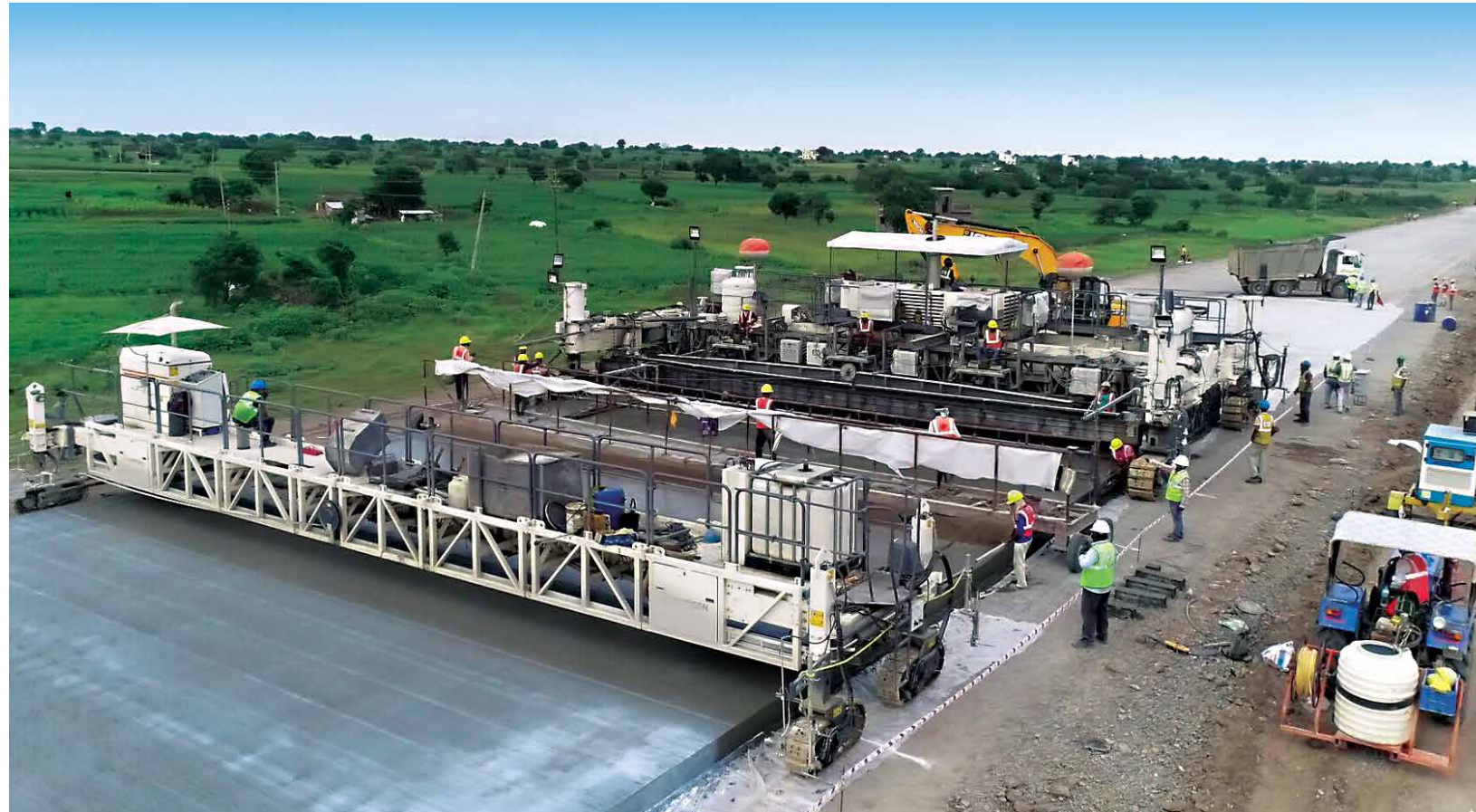
Pavement Quality Concreting at the Mumbai Nagpur Expressway Project
