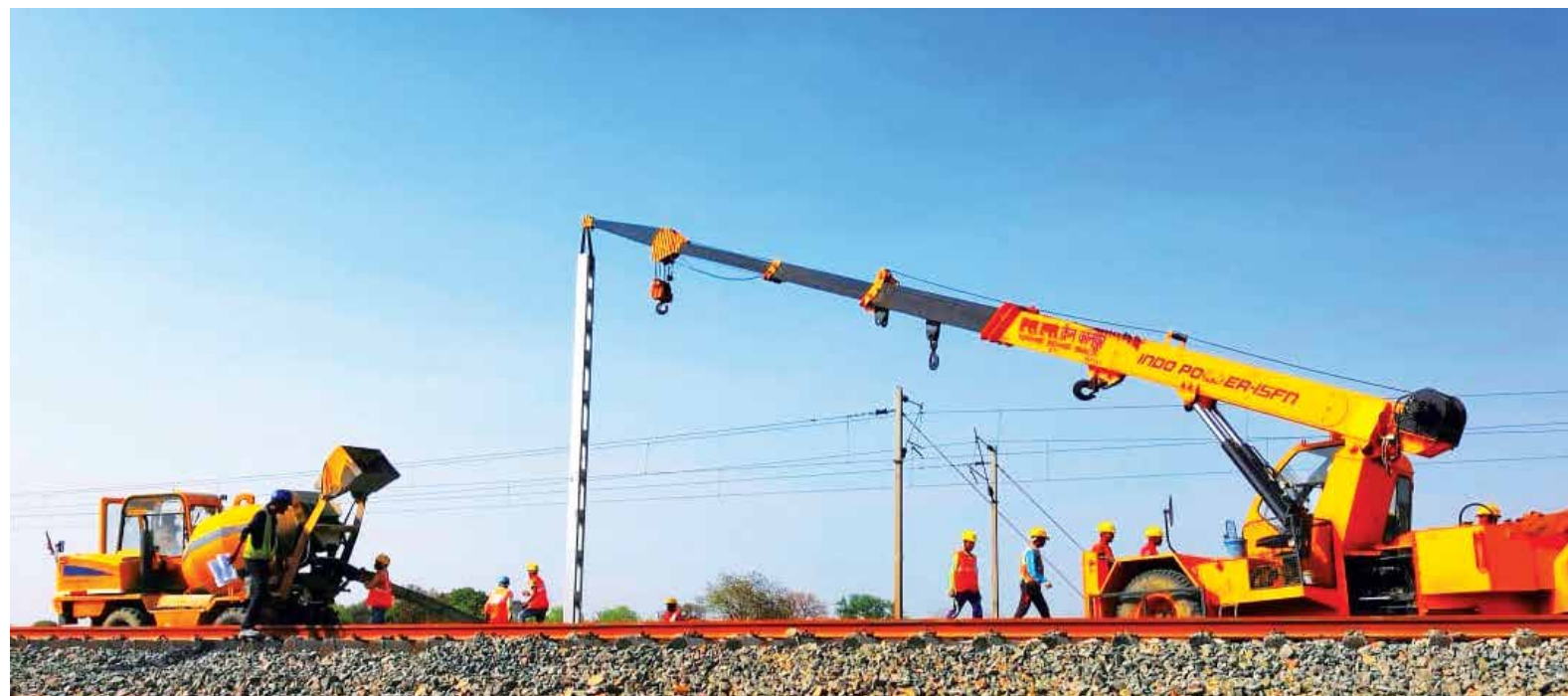
Erection of mast at CP 204
