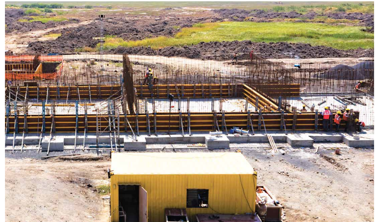
Lamella clarifier wall shuttering works at the 100 MLD Desalination Plant Project, Dahej
