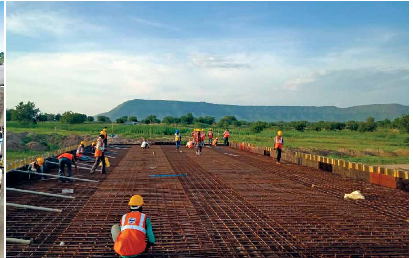
Reinforcement tying work at the Mumbai Nagpur Expressway Project
