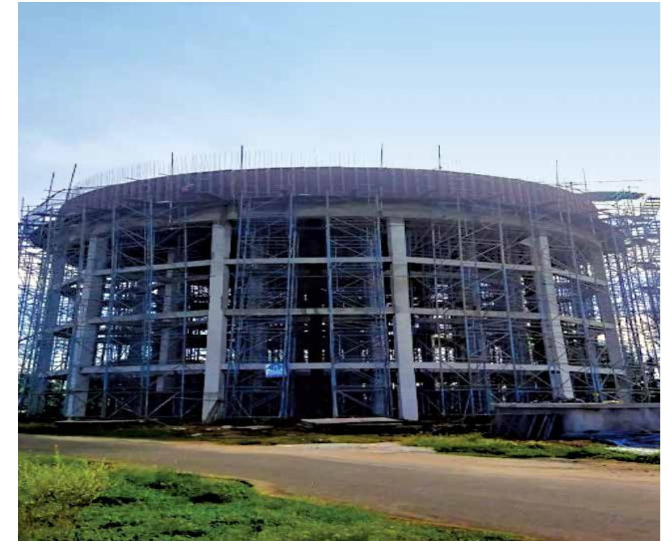
Elevated storage reservoir under construction at the Erode Water Supply Project
