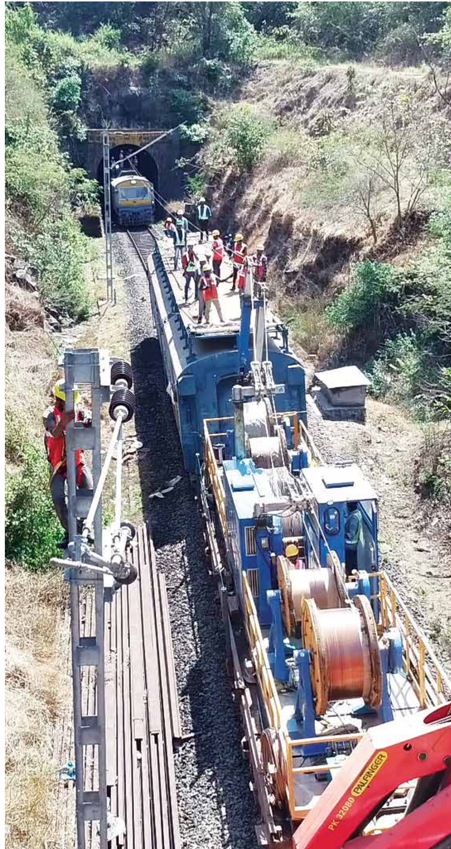
OHE stringing through automatic wiring train
