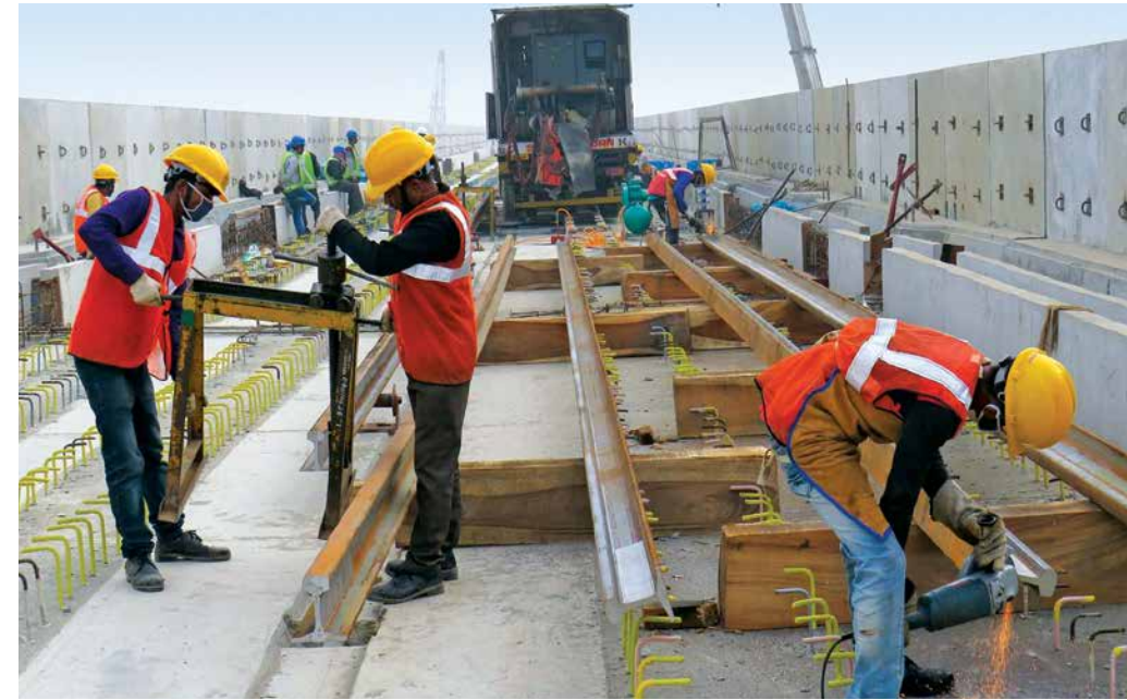
Ballastless trackworks at Dhaka Metro Project
