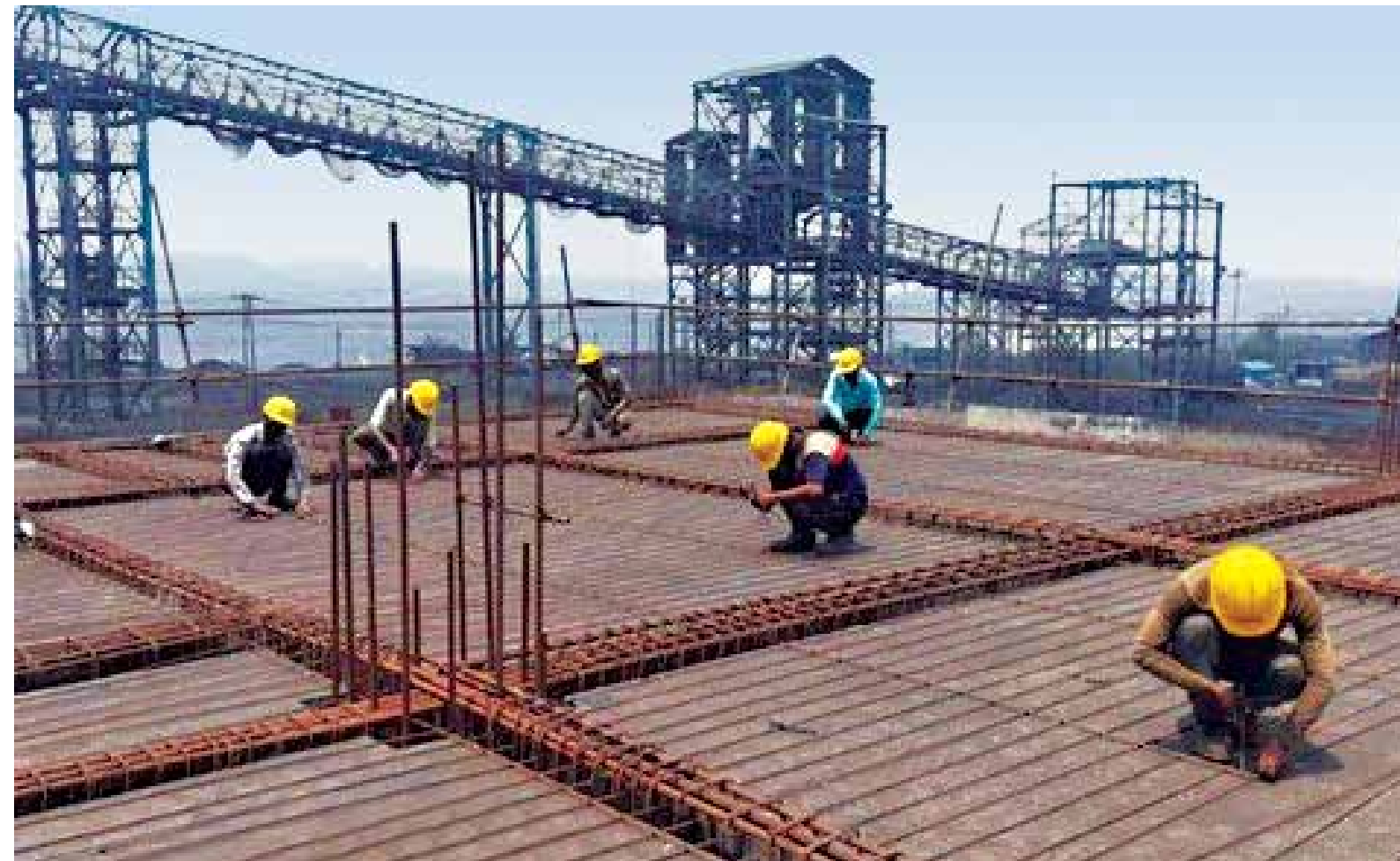
Civil work proceeding at the MCL - Bhubaneswari project with social distancing
