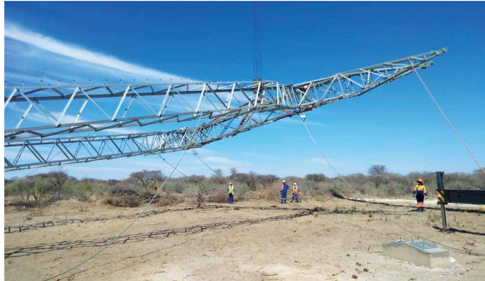
Tower erection at 400 kV Morepule B–Orapa–Mawana Project, Botswana
