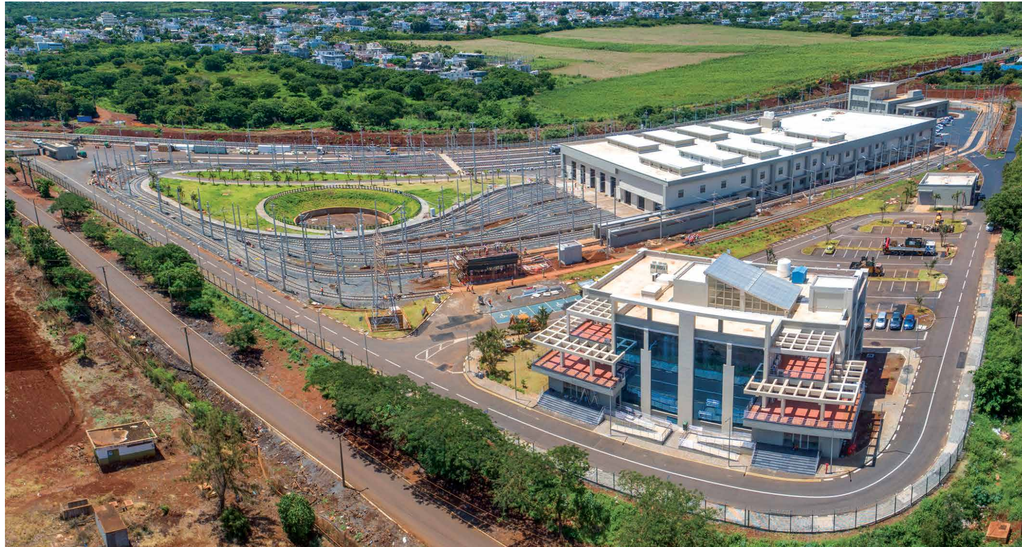
Aerial view of Mauritius Metro Depot
