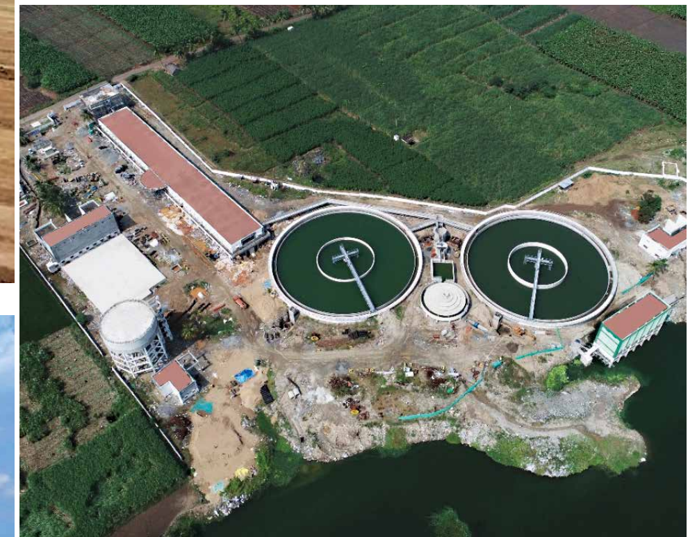
Overview of the Erode Water Supply Project
