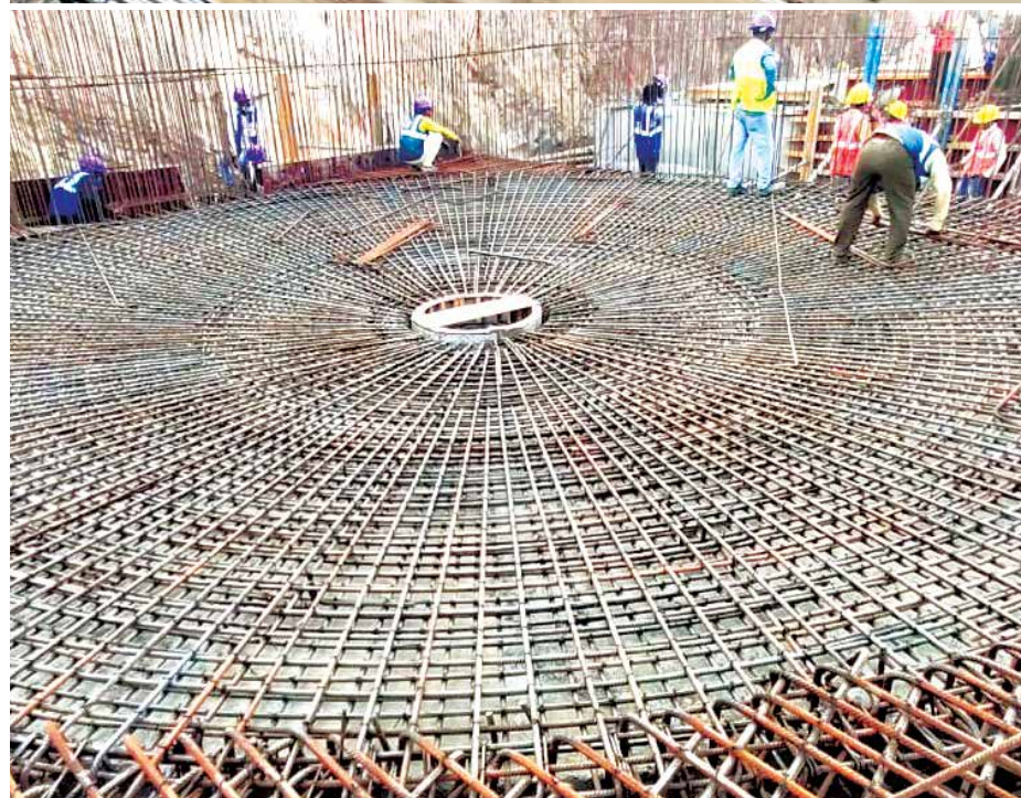
Tube Settler bar binding works at Udaipur Integrated Infrastructure Project
