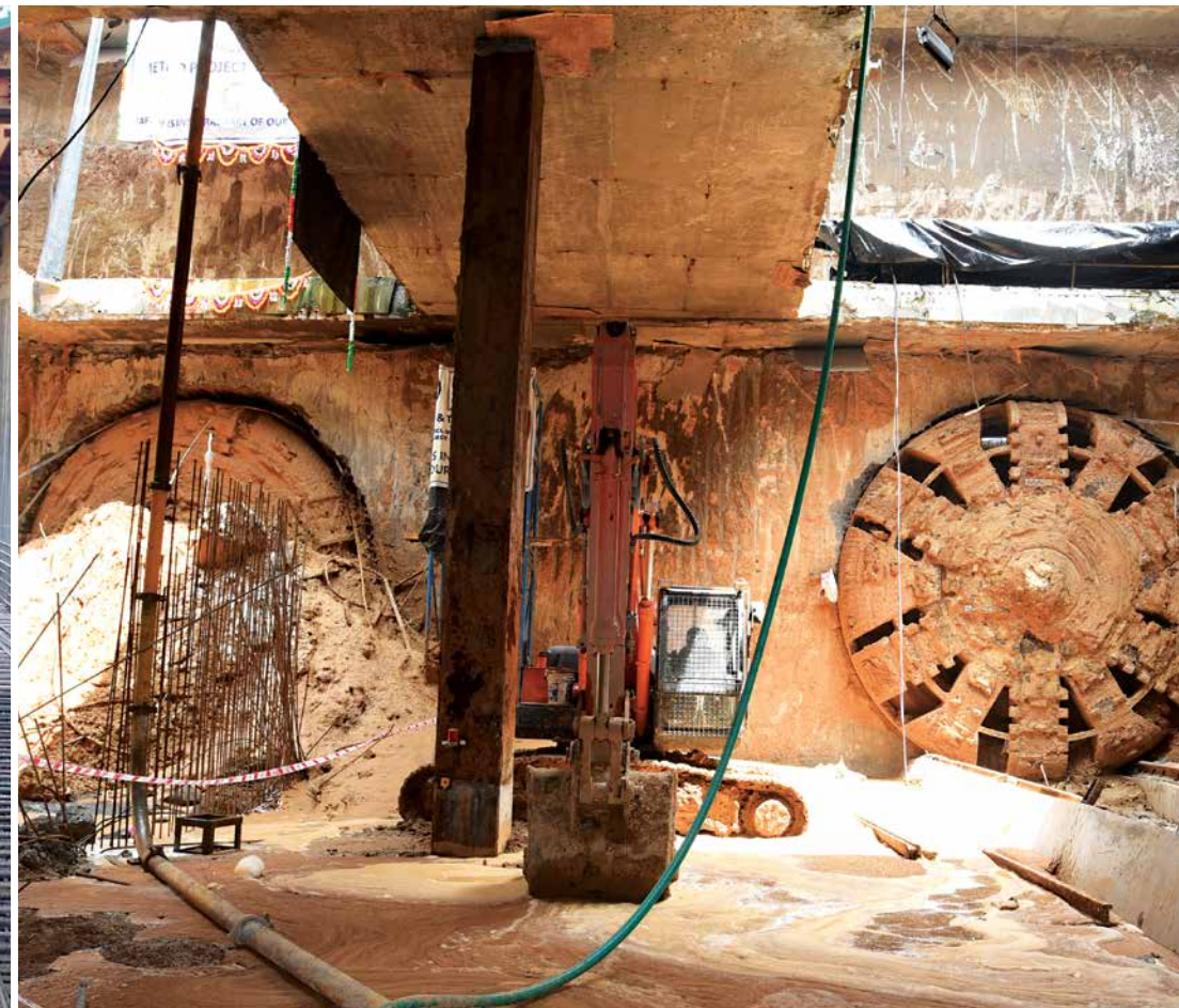
Completion of TBM tunnelling at Ahmedabad Metro
