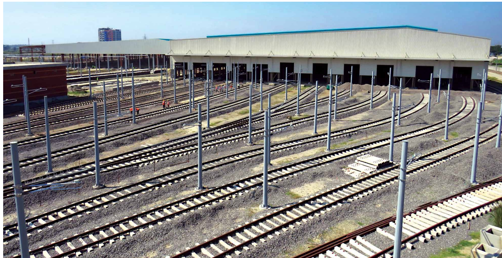
Completed section of trackworks at Dhaka Metro Depot
