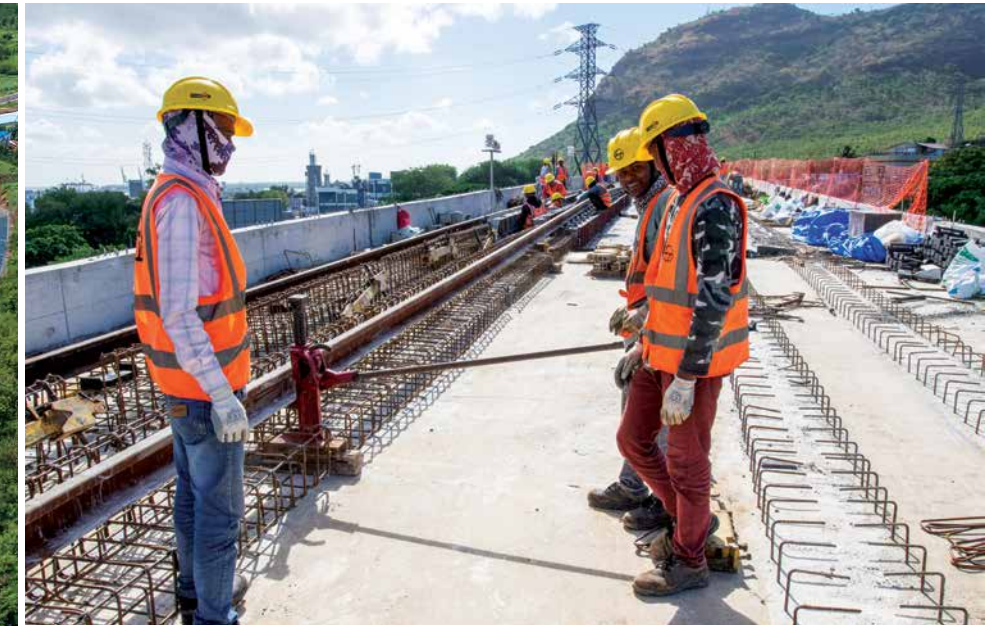
Plinth trackworks at Mauritius LRT
