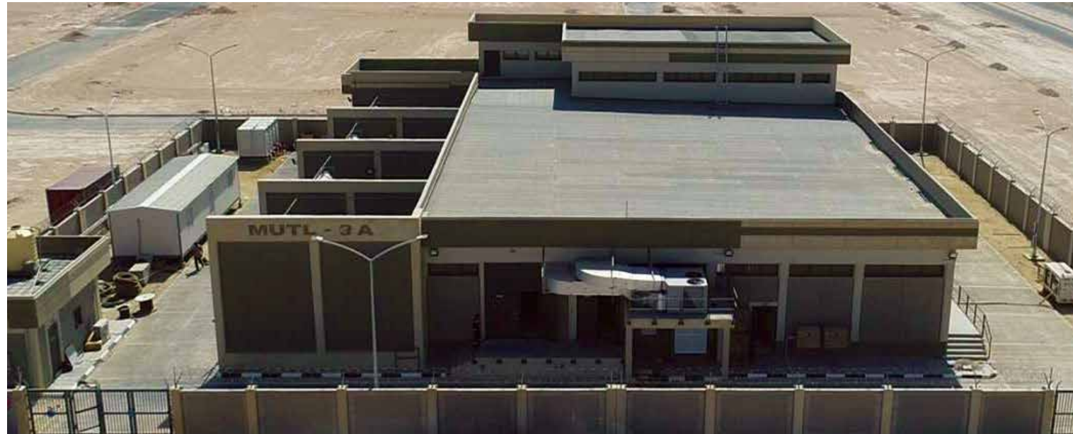
Overall view of the PAHW Substation, Kuwait
