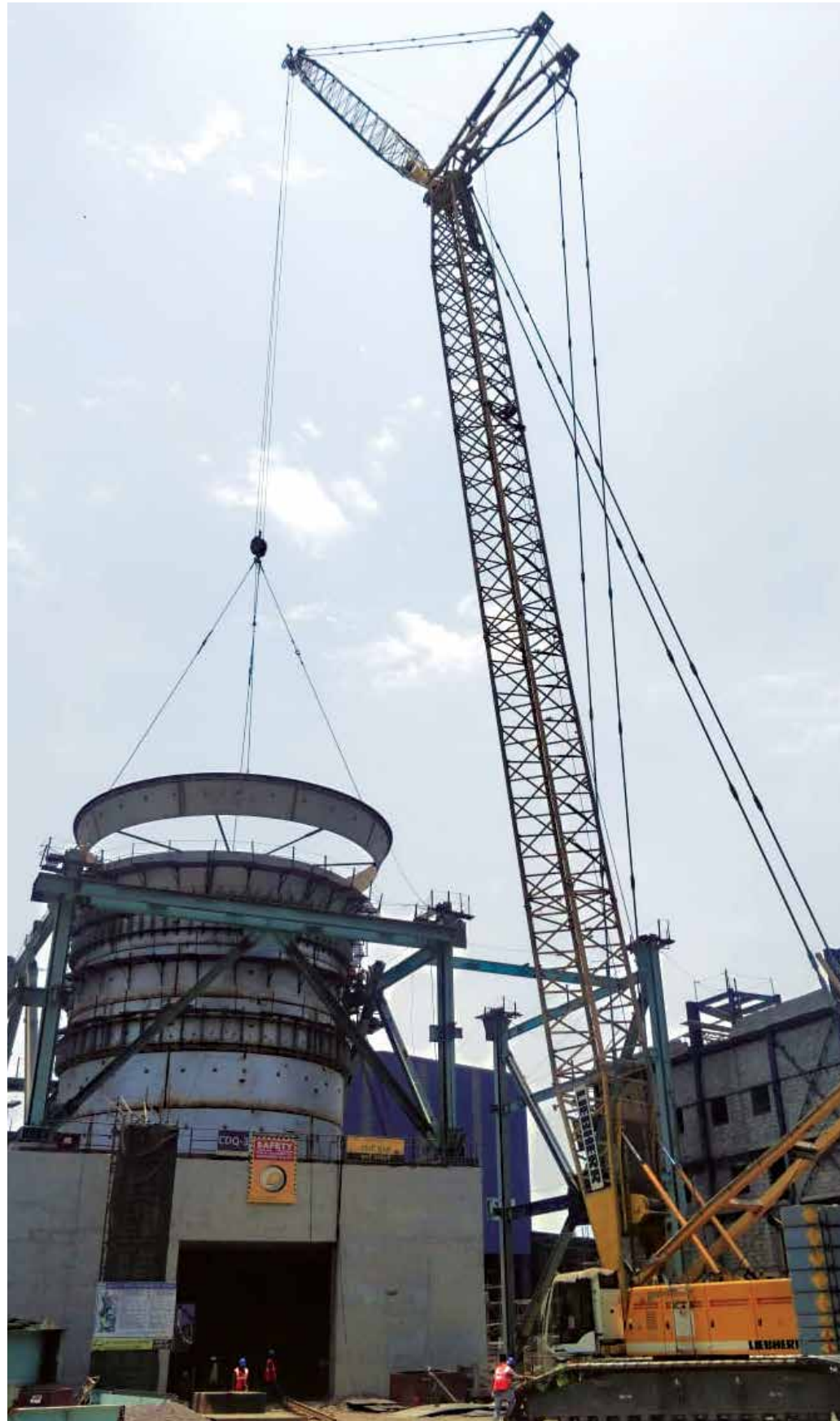
Erection of main chamber shell at CDQ 3, JSW, Dolvi project
