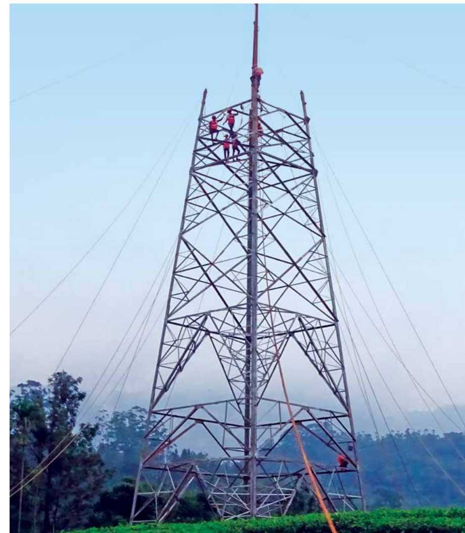
Tower erection at the 220/110 kV Kochi Transmission Line Project
