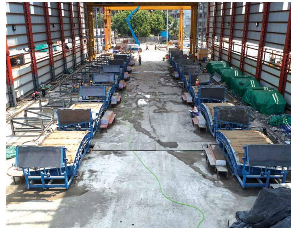
Precast Segment Casting Yard at MCRP Package - 4
