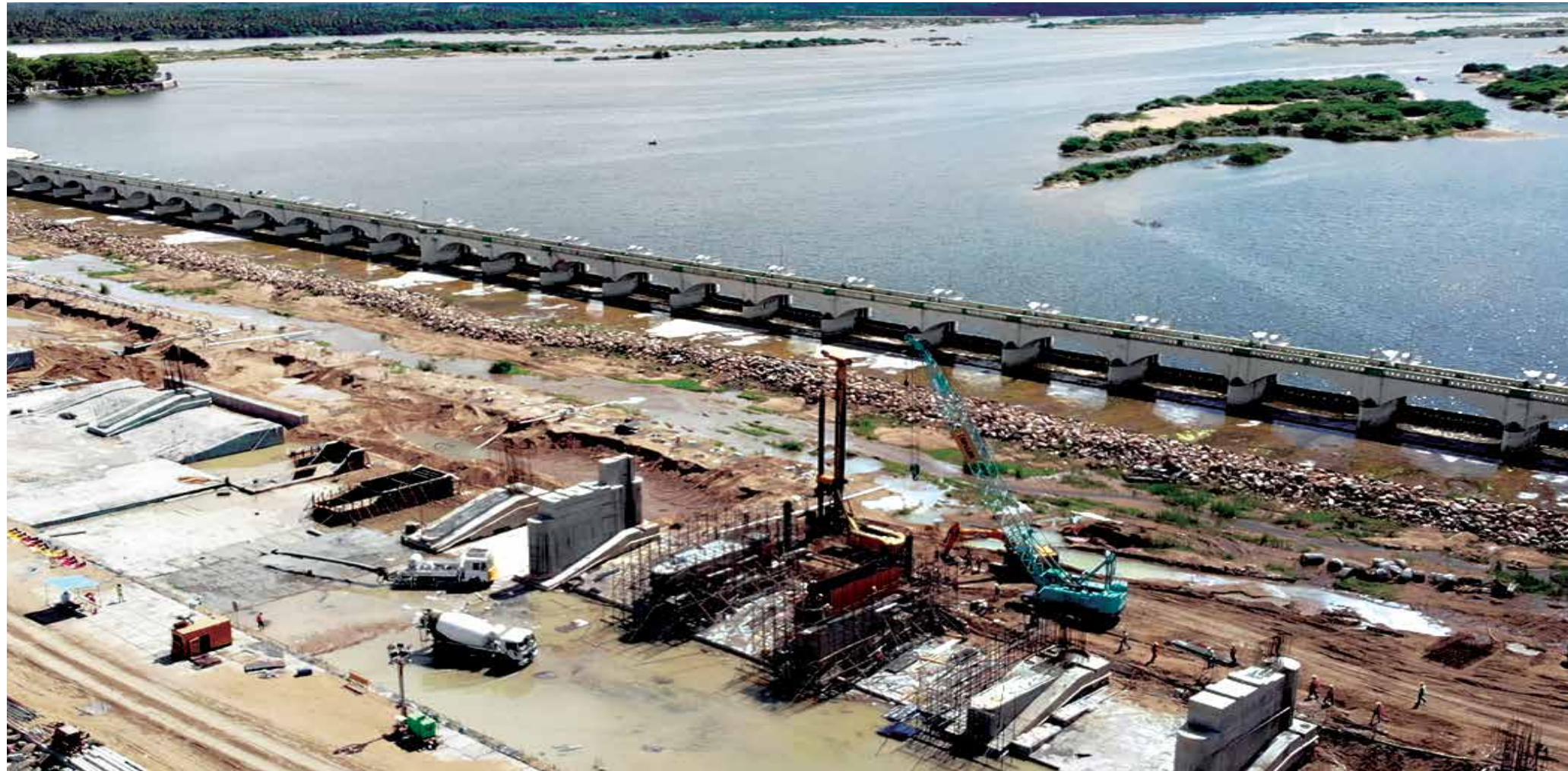
Civil works at Mukkombu Upper Anaicut Barrage Project
