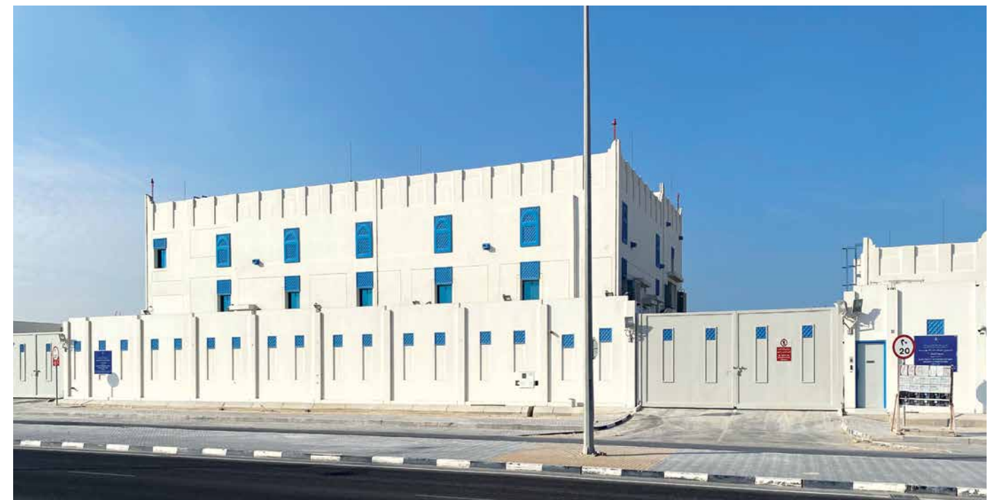
132/11 kV Mashaf-2 Substation
