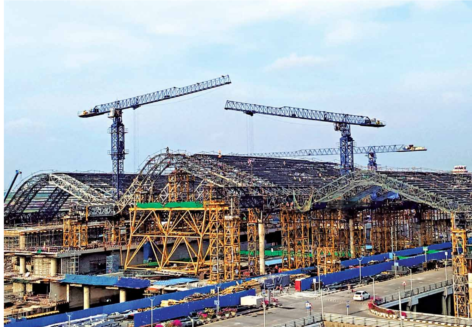
Chennai International Airport
