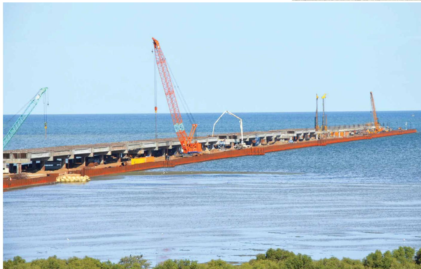
Seawater intake outfall structure at Uppur
