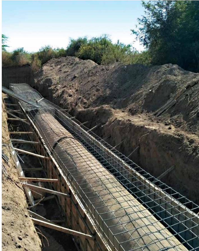
Pipe encasing for river crossing
