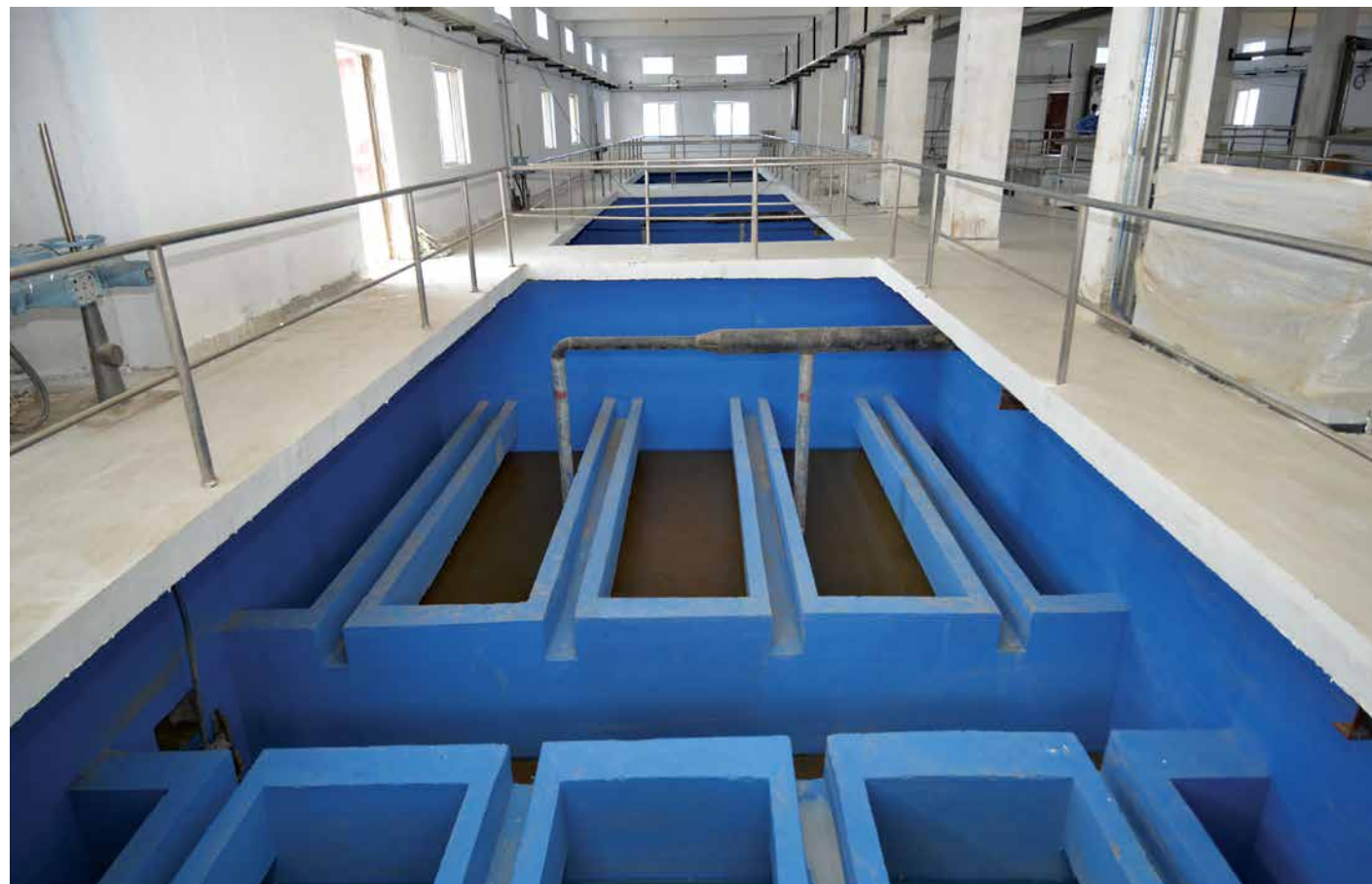
Rapid gravity sand filter beds
