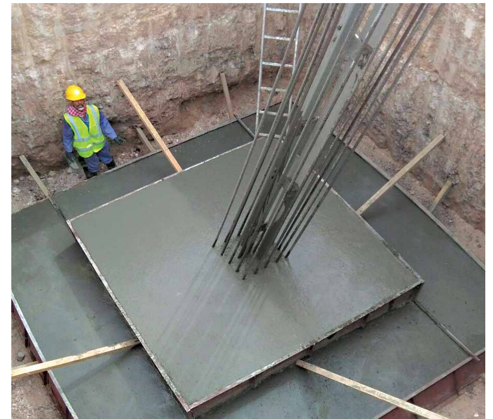
Completion of pad 1 & 2 concreting for tower foundation
