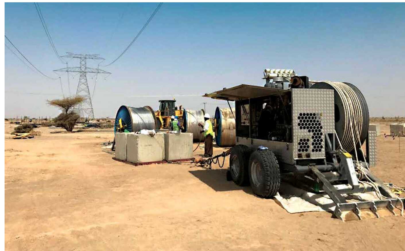
Stringing work in progress
