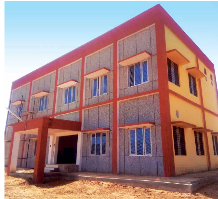
Master Control Center
