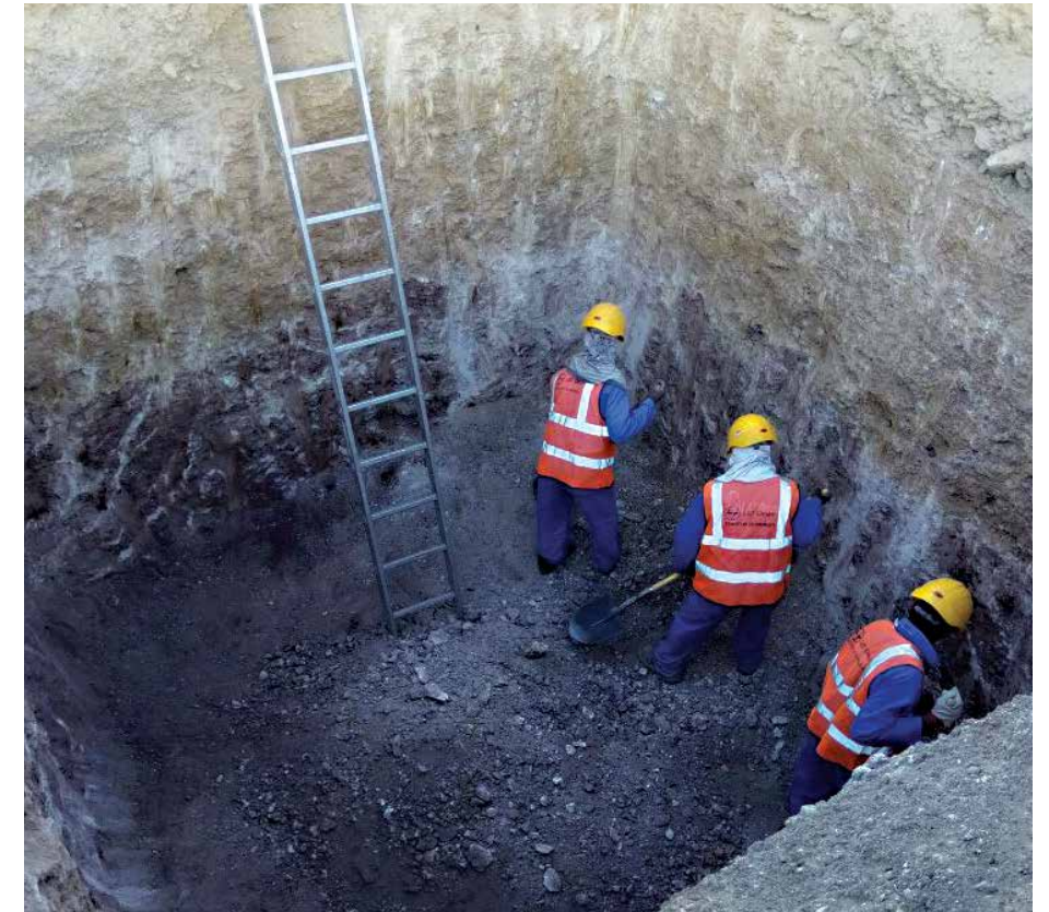
Pit dressing in progress for tower foundation
