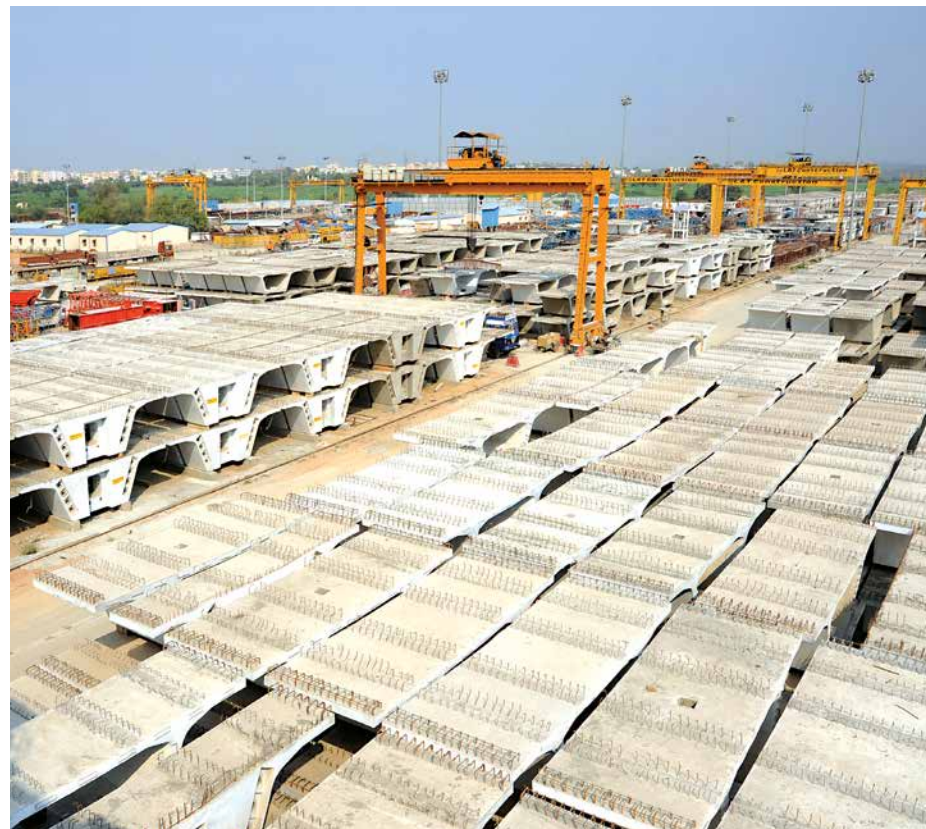
One of the largest precast yard in Asia
