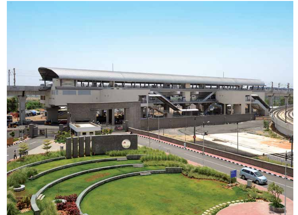
A picturesque view of metro station
