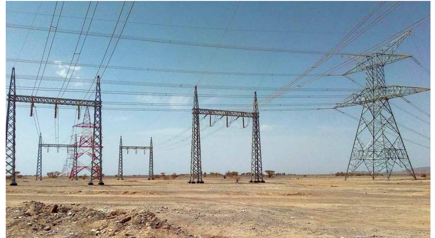
Lowering of existing 132 kV OHL using underpass gantries to cross 400 kV OHL
