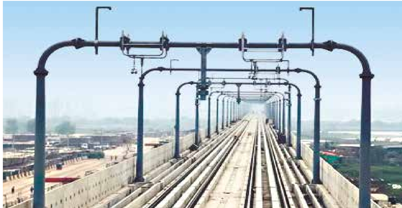
Masts for DC Overhead Catenary System
