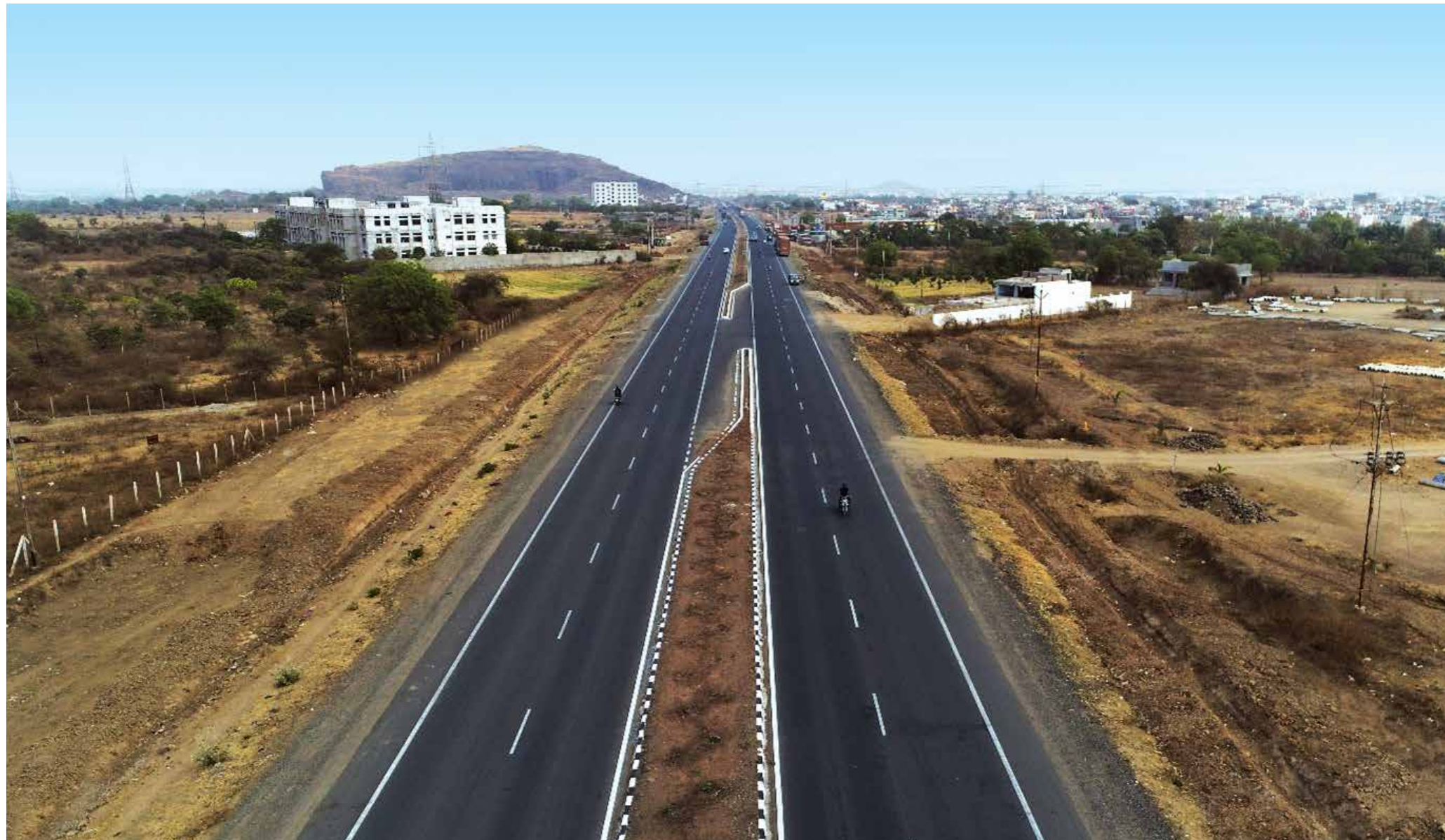
4 lanes completed from CH 304+000 to CH 305+000 in the middle of a forest area
