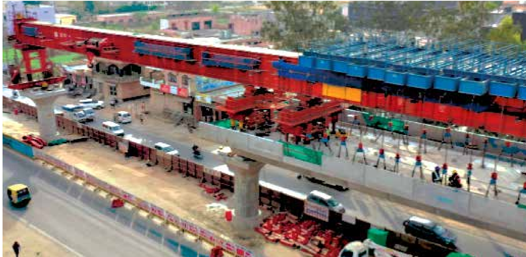
Launching girders at the RRTS project
