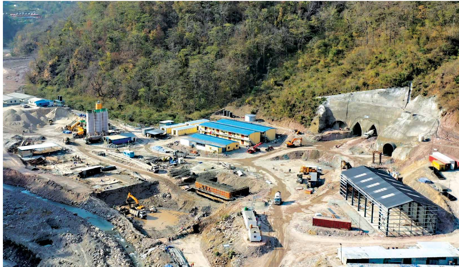
RVNL Pkg 2 - Site Camp and Tunnel Portals
