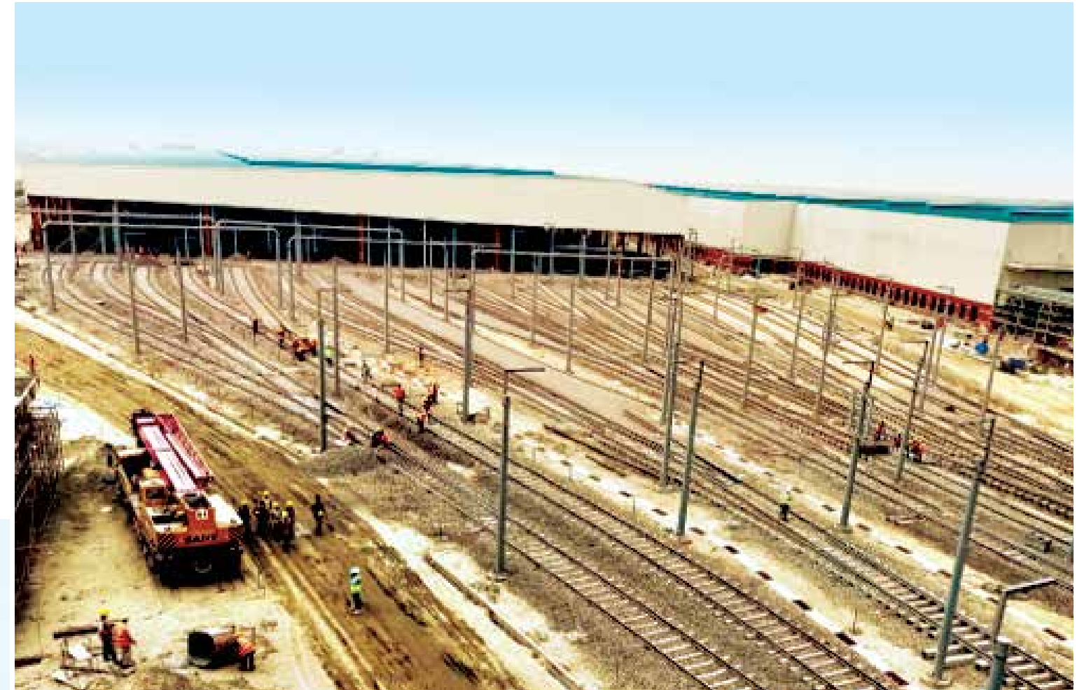
Phase 2 works: outside stabling shed
