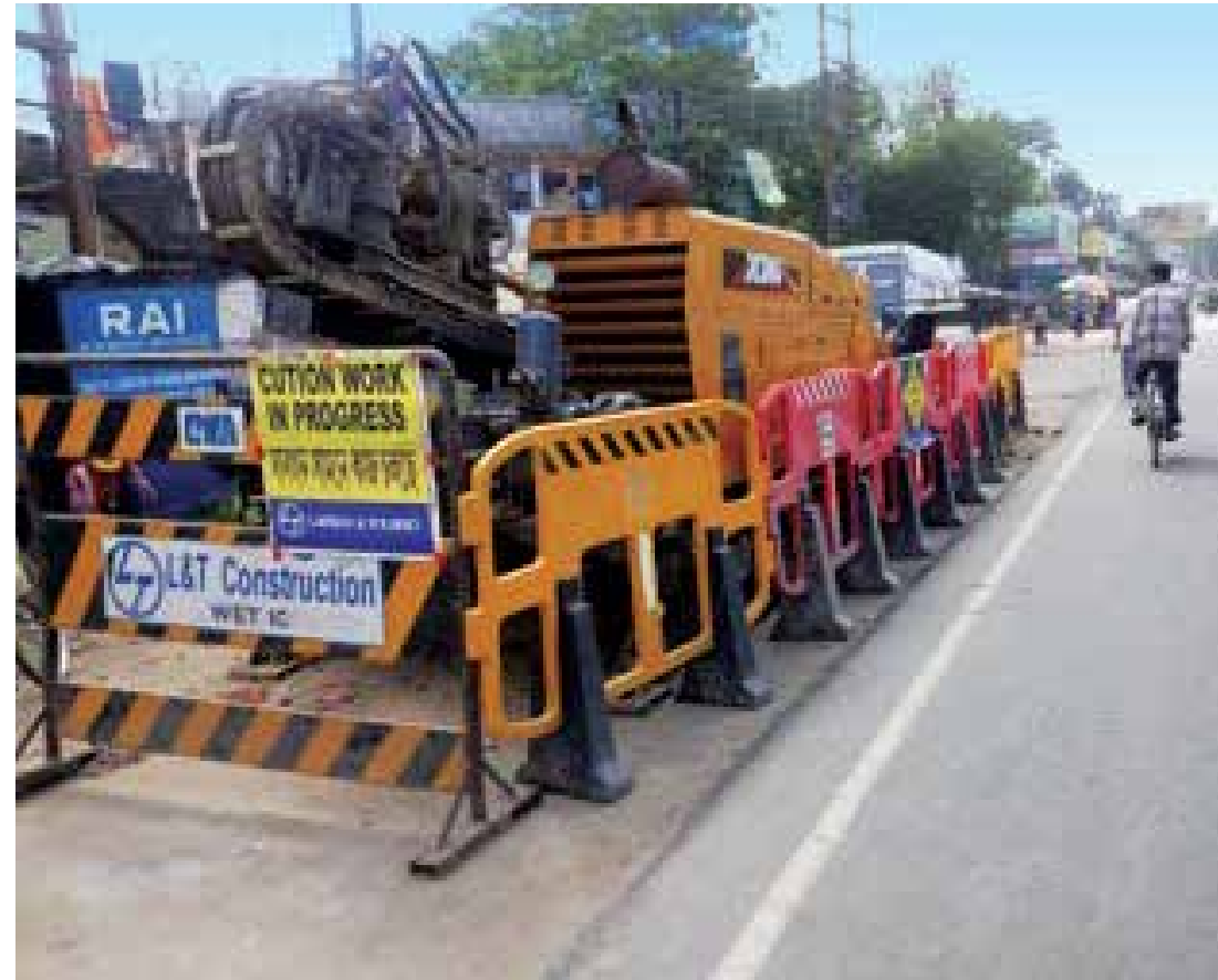
Horizontal drilling machine deployed at Barrackpore Integrated Sewerage System Project
