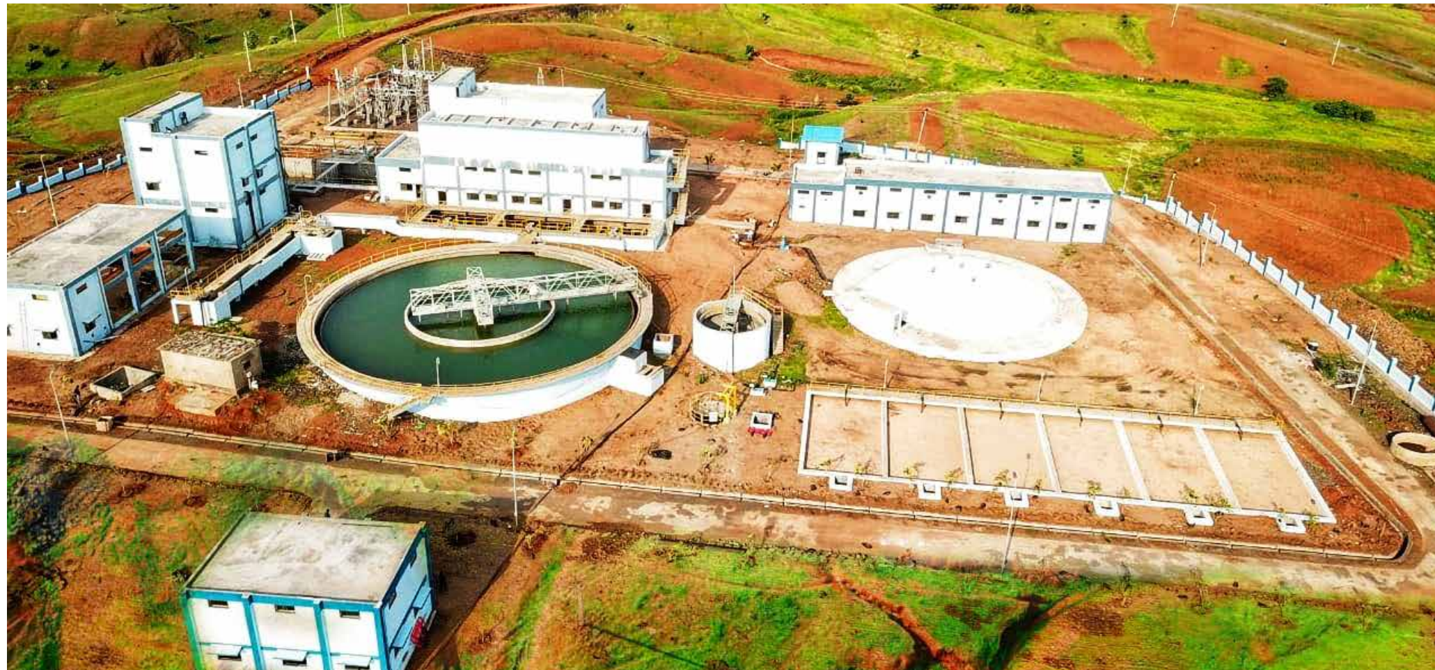
Overview of the 18.6 MLD Water Treatment Plant
