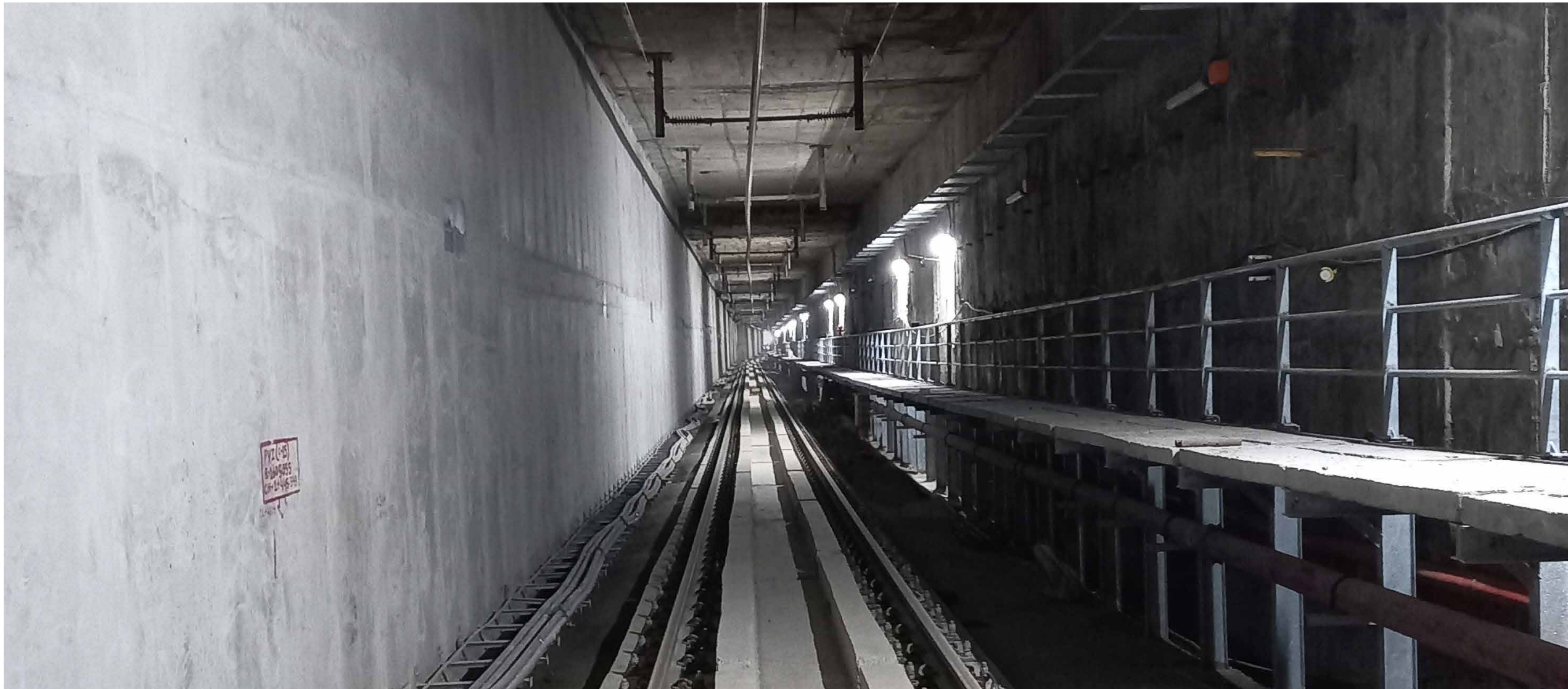
View of the cut and cover tunnel at Tondiarpet, CMRL
