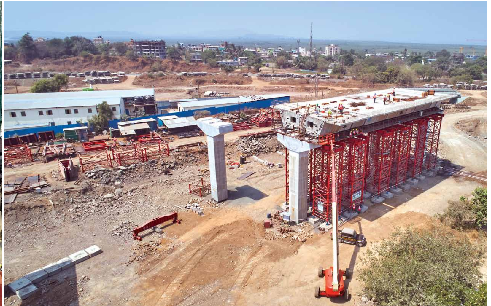
MTHL 3 - Span Erection
