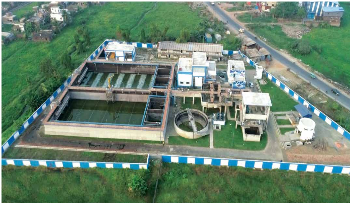
18 MLD Sewerage Treatment Plant at Barrackpore
