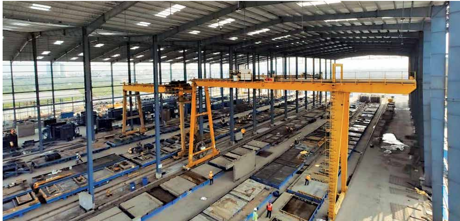
Precast Yard – CIDCO, Navi Mumbai
