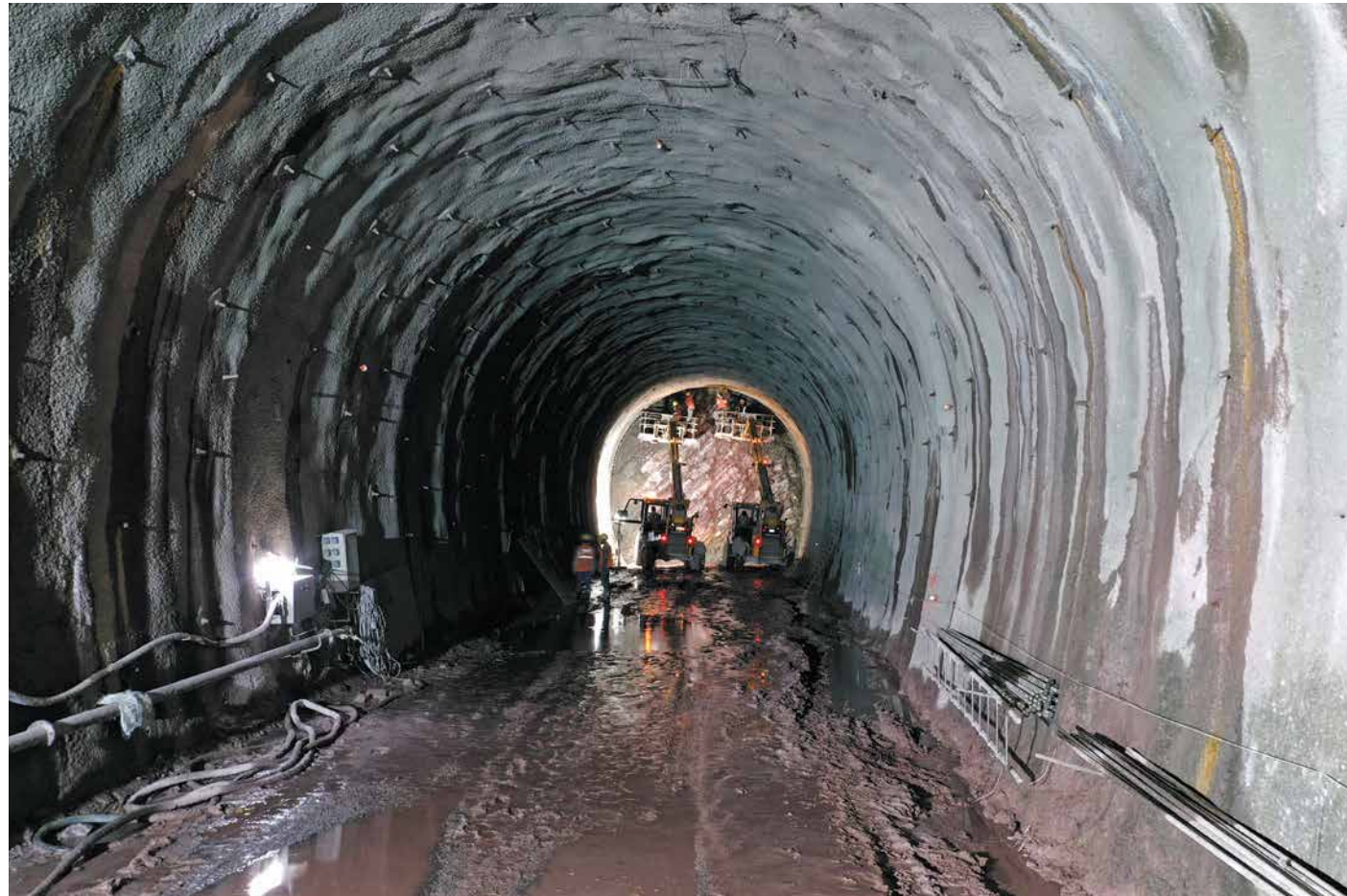
Tunnel excavations in progress
