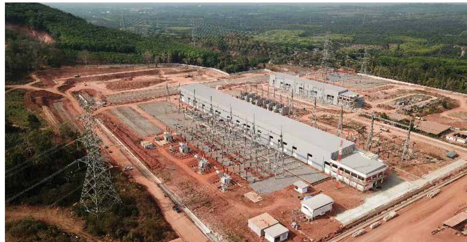
500/230 kV Surat Thani-2 GIS under construction
