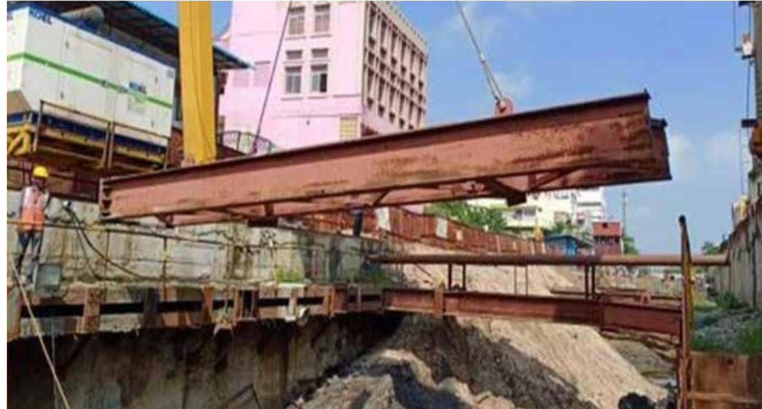
Cut and cover at Tondiarpet, CMRL
