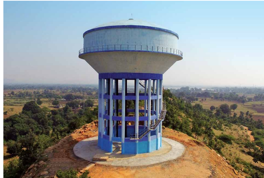
1150 KL Overhead Service Reservoir at Banswara-Pratapgarh WSS
