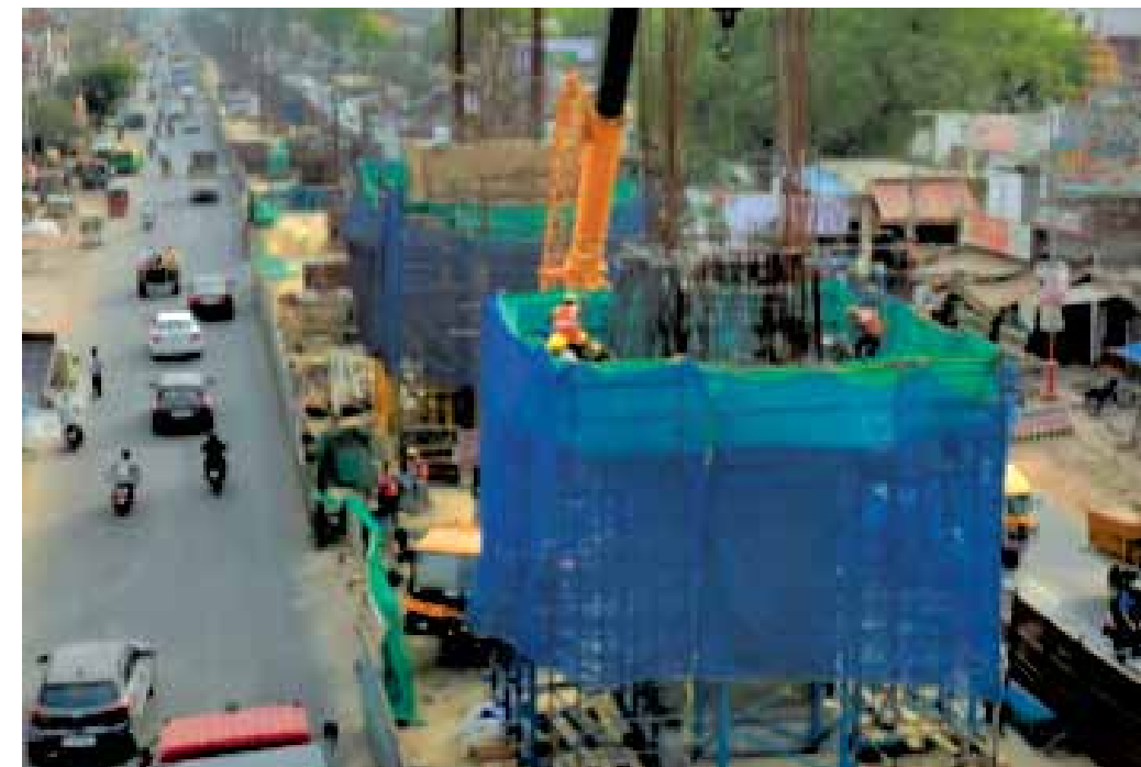
Pier works at RRTS
