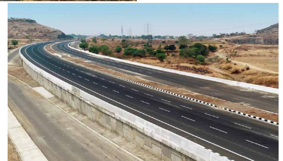
Another completed 4-lane stretch with a median opening
