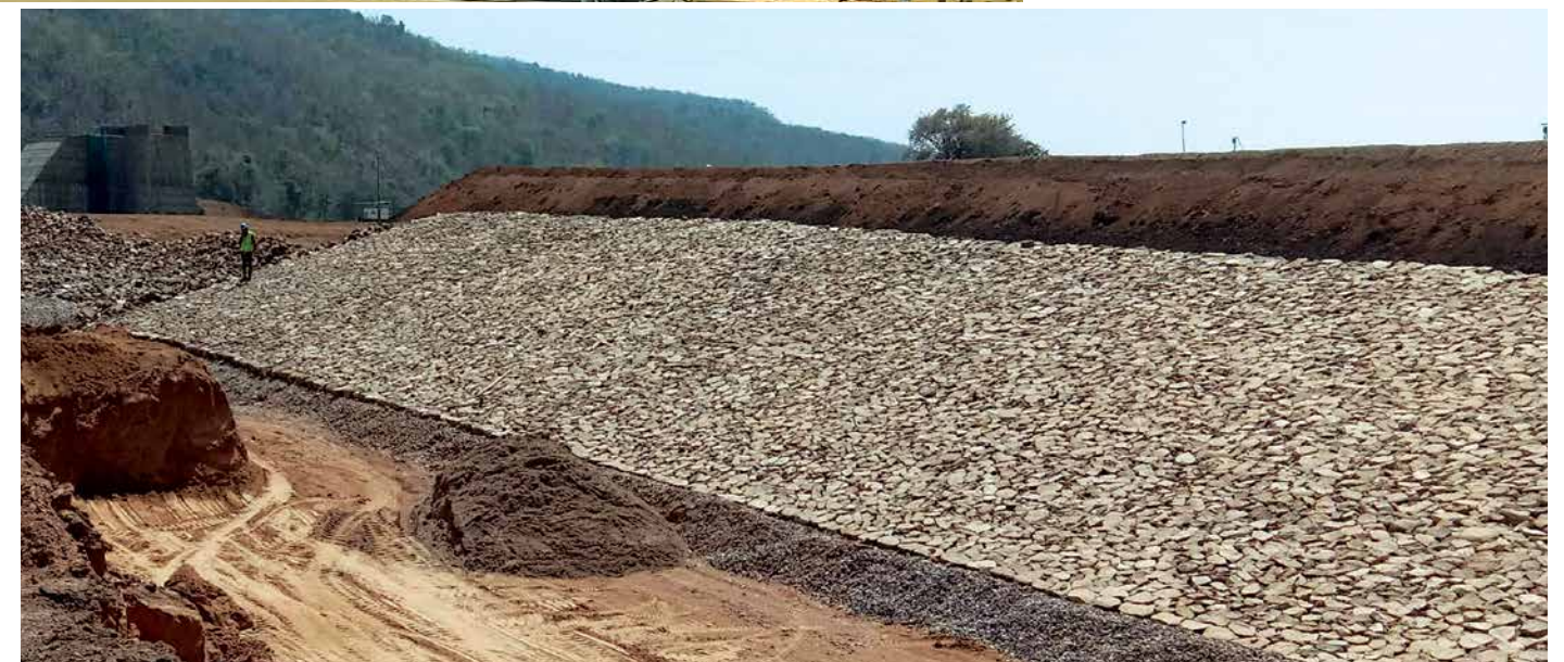
Stone pitching works at Runj dam, M.P.
