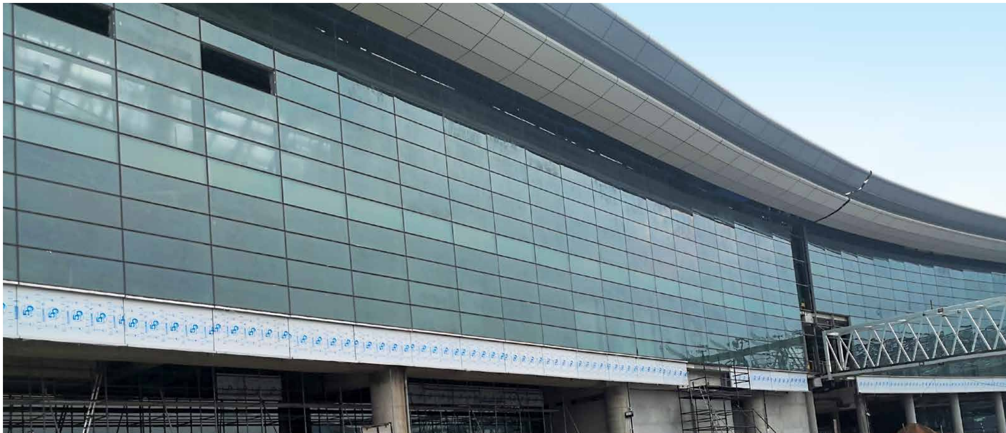
Hyderabad International Airport Expansion Project
