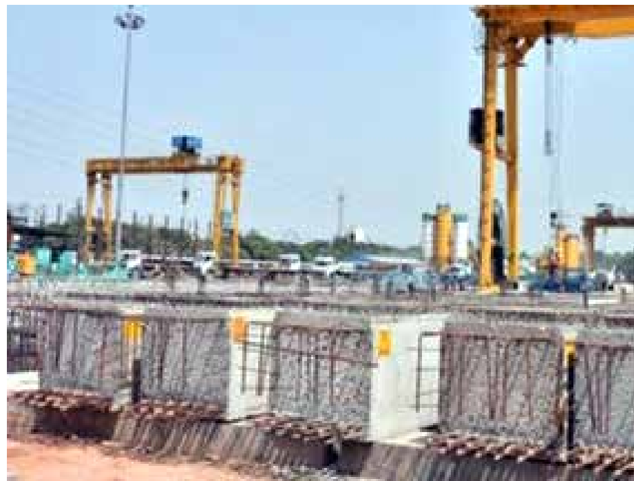
Precast yard set up
