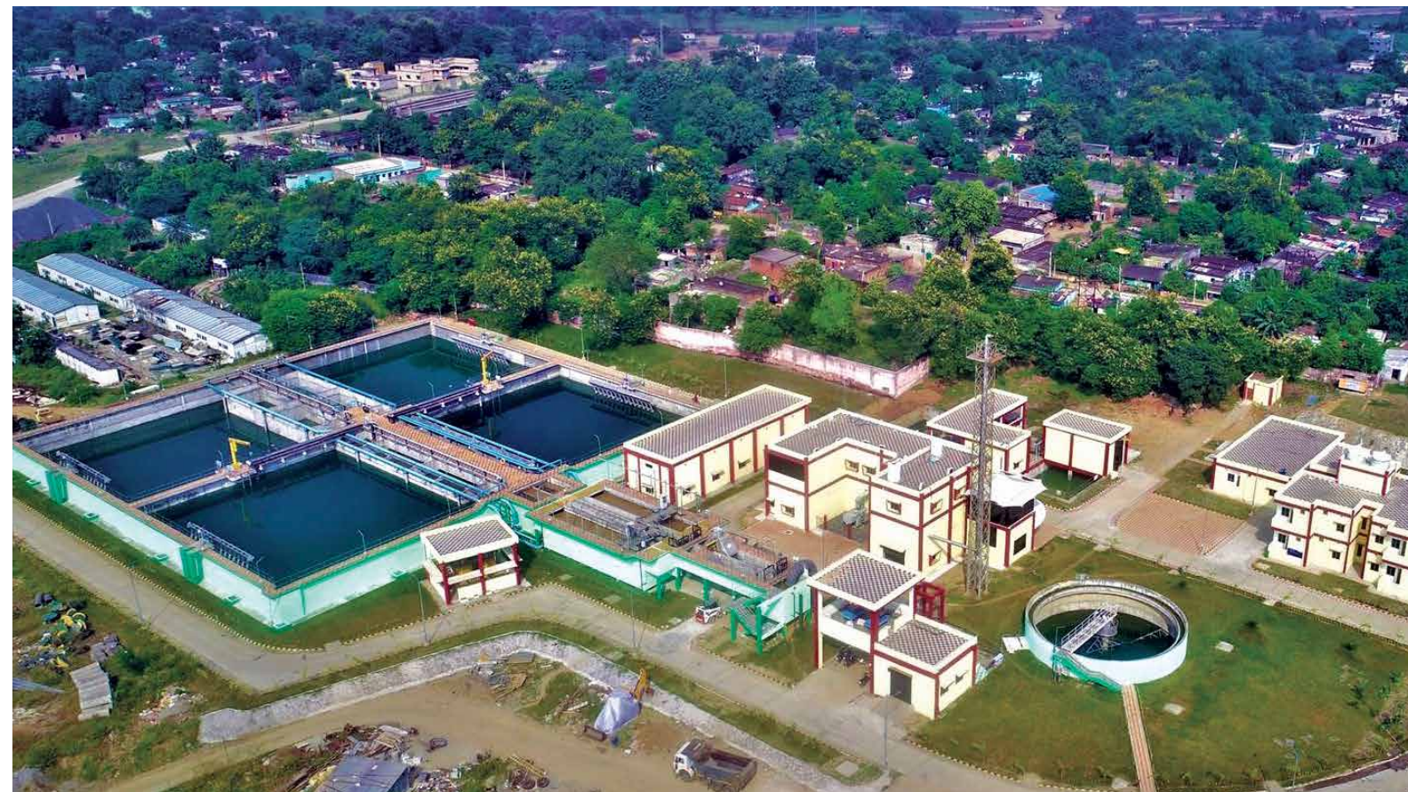
40 MLD Sewerage Treatment Plant at Rourkela
