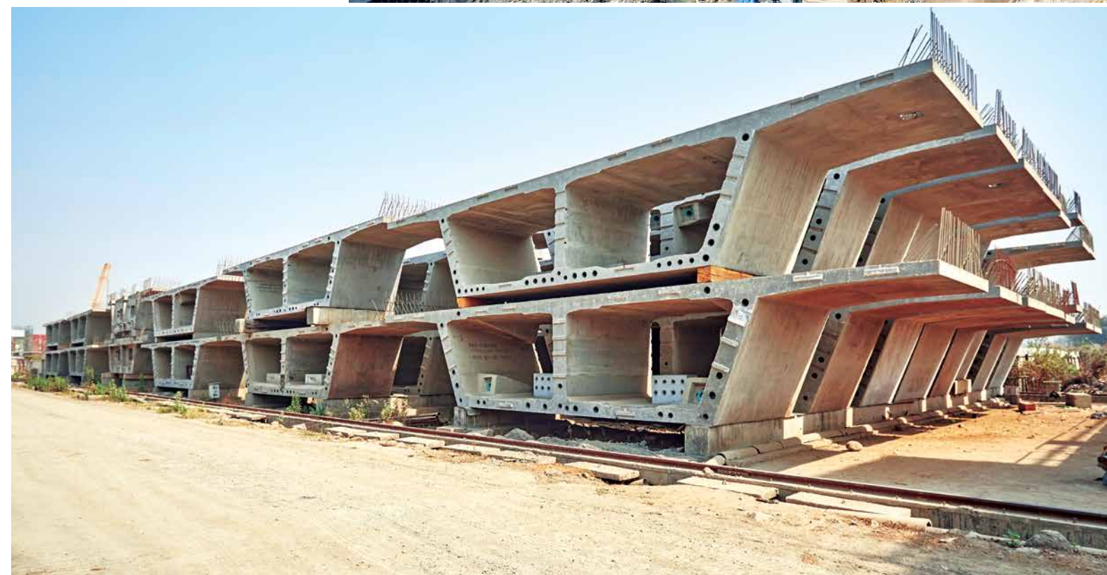
Precast elements stacked in the precast yard at MTHL Pkg 3
