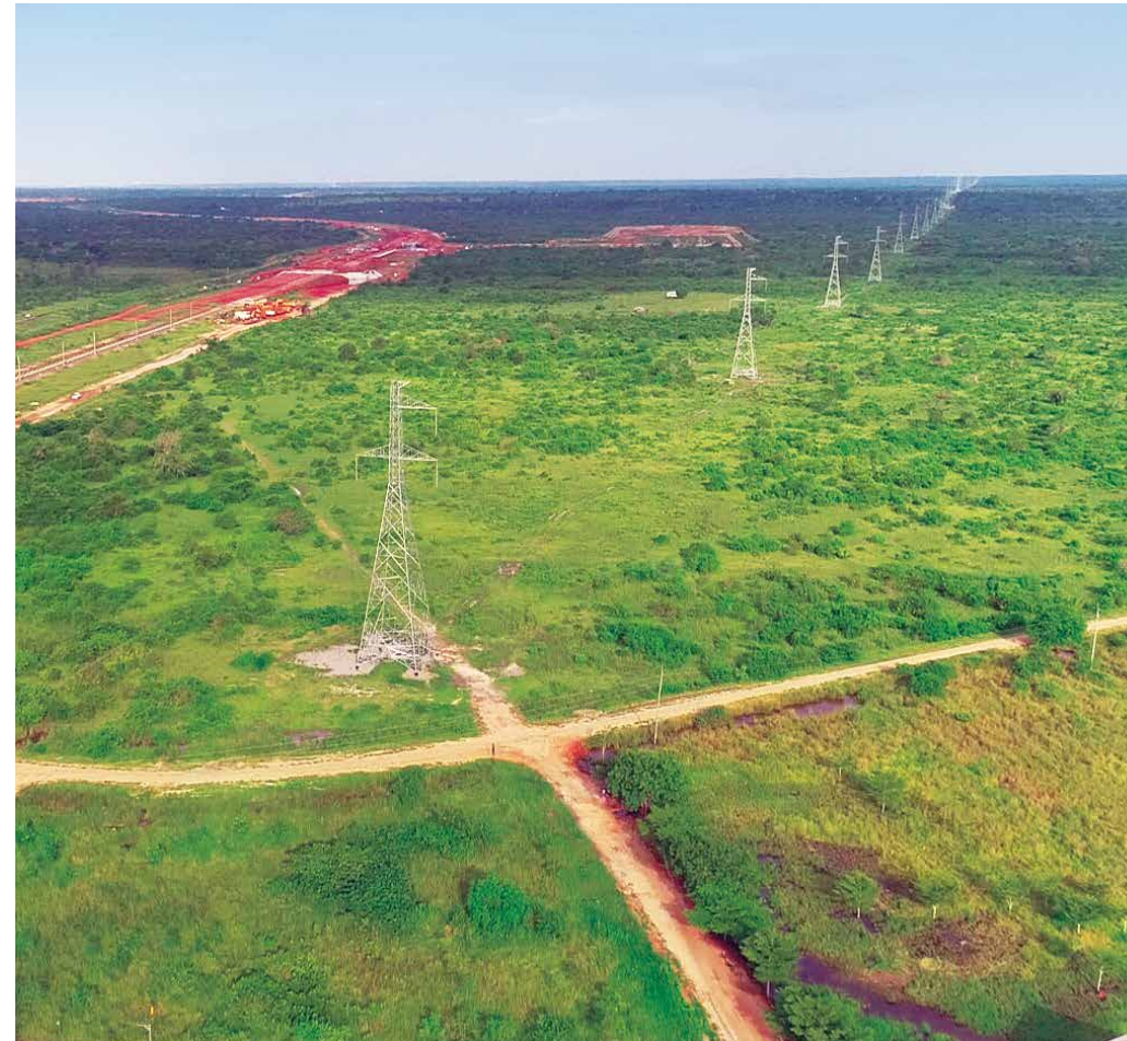
220 kV Single Circuit Transmission Line, Tanzania
