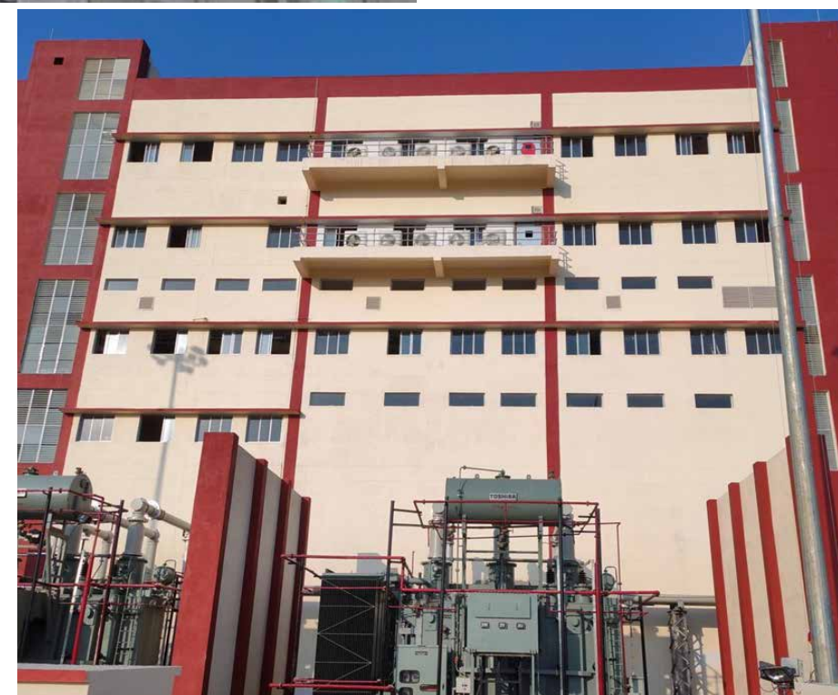
Ground plus 6 floor control building of the GIS at Ranchi
