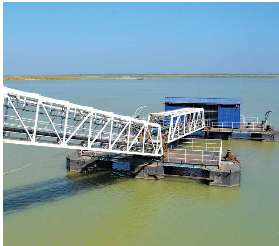
Floating barge intake at Sahibganj, Jharkhand
