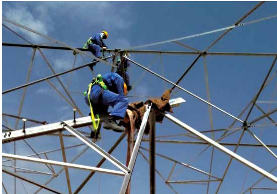
Scaling heights with secure rope grab fall arrestors
