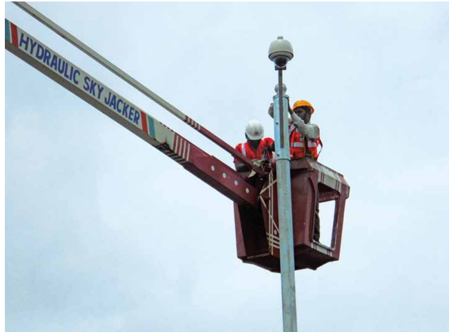
Workmen fixing a surveillance camera
