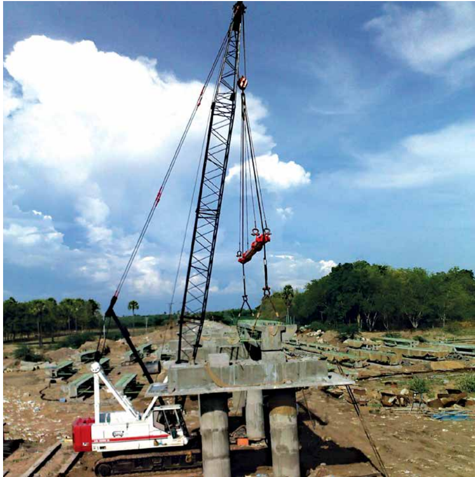
A TFC 280-75 T crane in action
