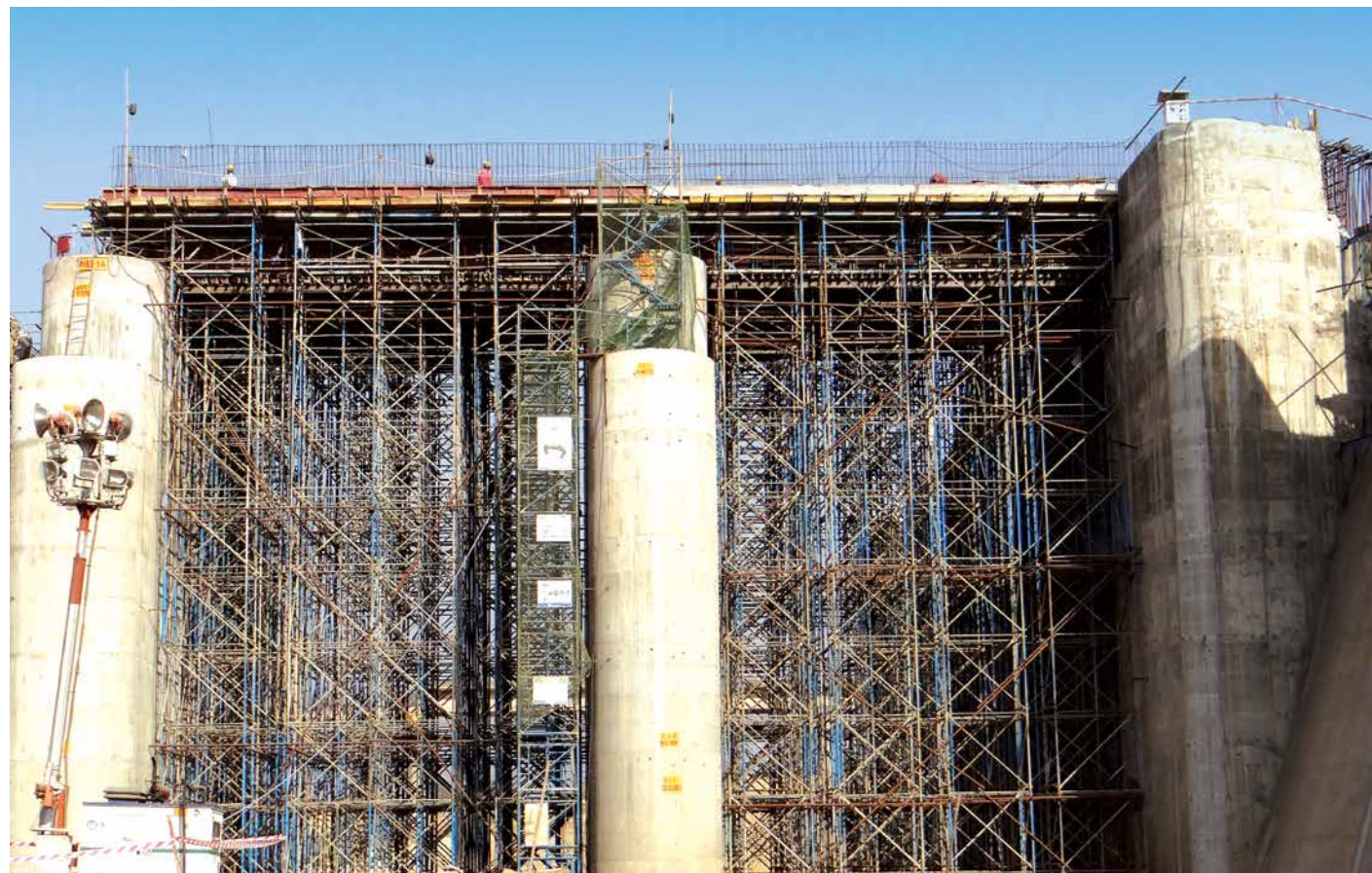
Scaffolding when building the Kharkai Barrage
