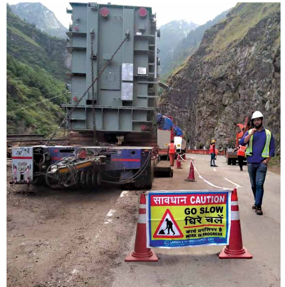
Safety messaging for public during the movement of hulking transformers
