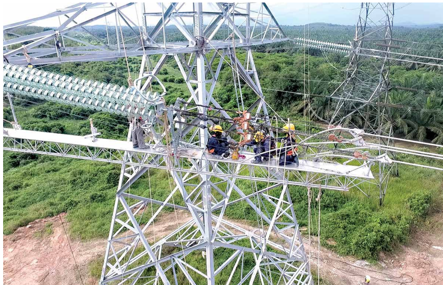
A safe platform on sag bridges for transmission tower erections
