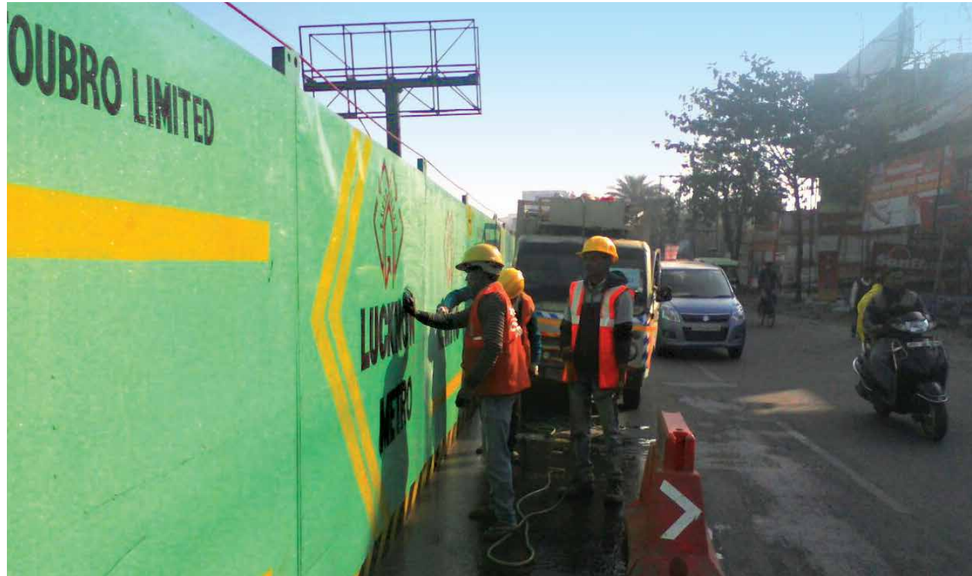
Communicating the message of safety
