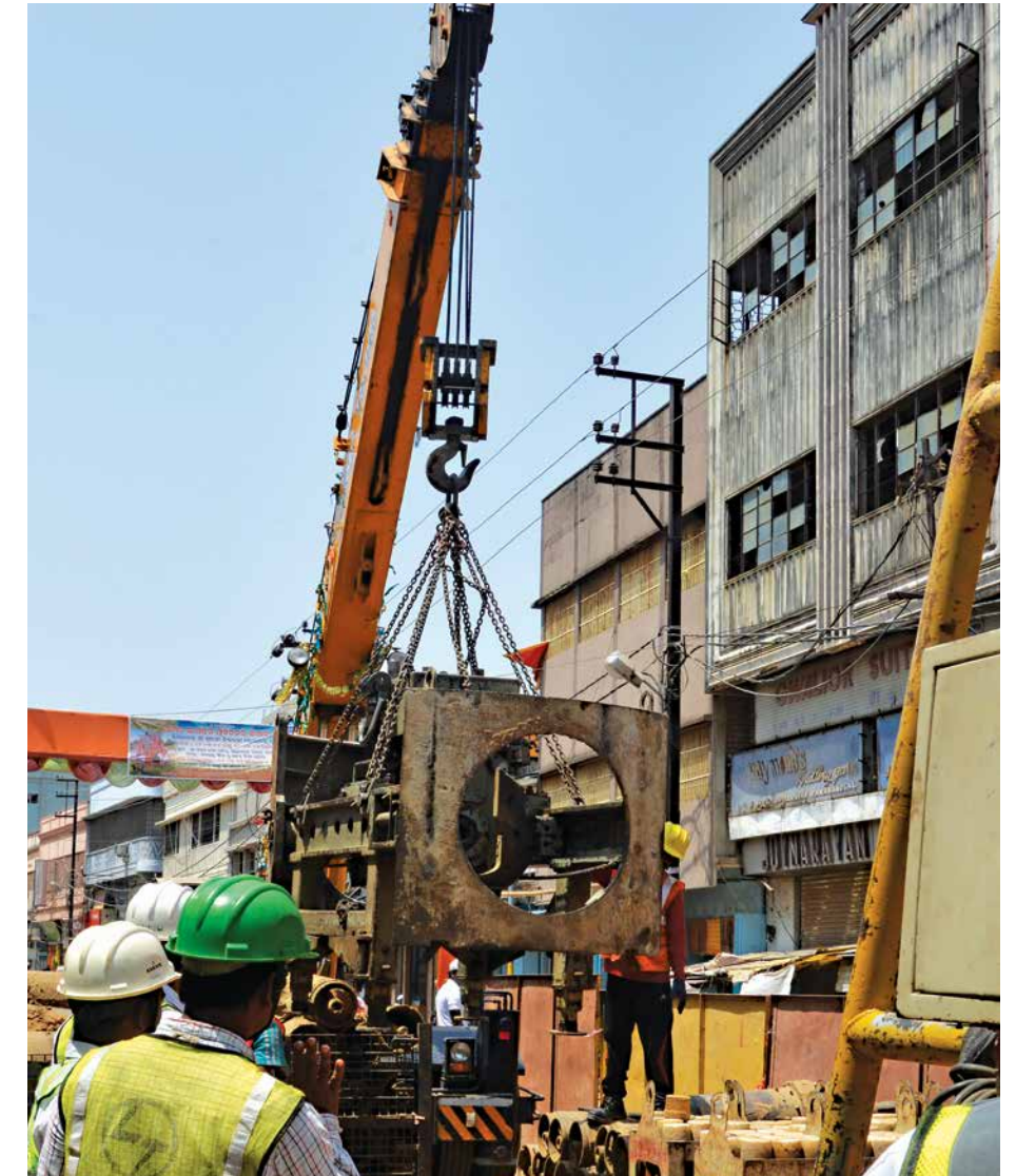
Precast duct installed at a sewage pipeline project
