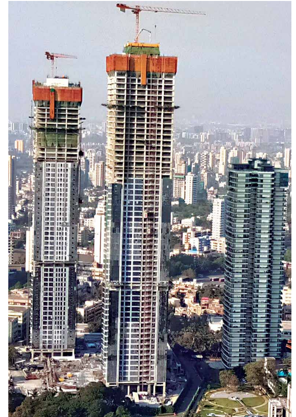
Creating a safe work environment at height
