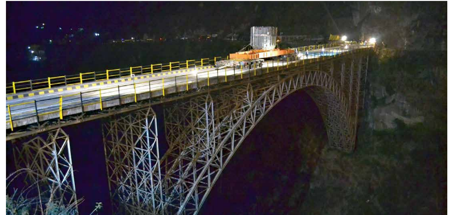
Safely moving a hulking transformer across an old bridge
