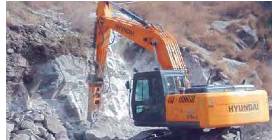
Rock breaker deployed for breaking hard rock
