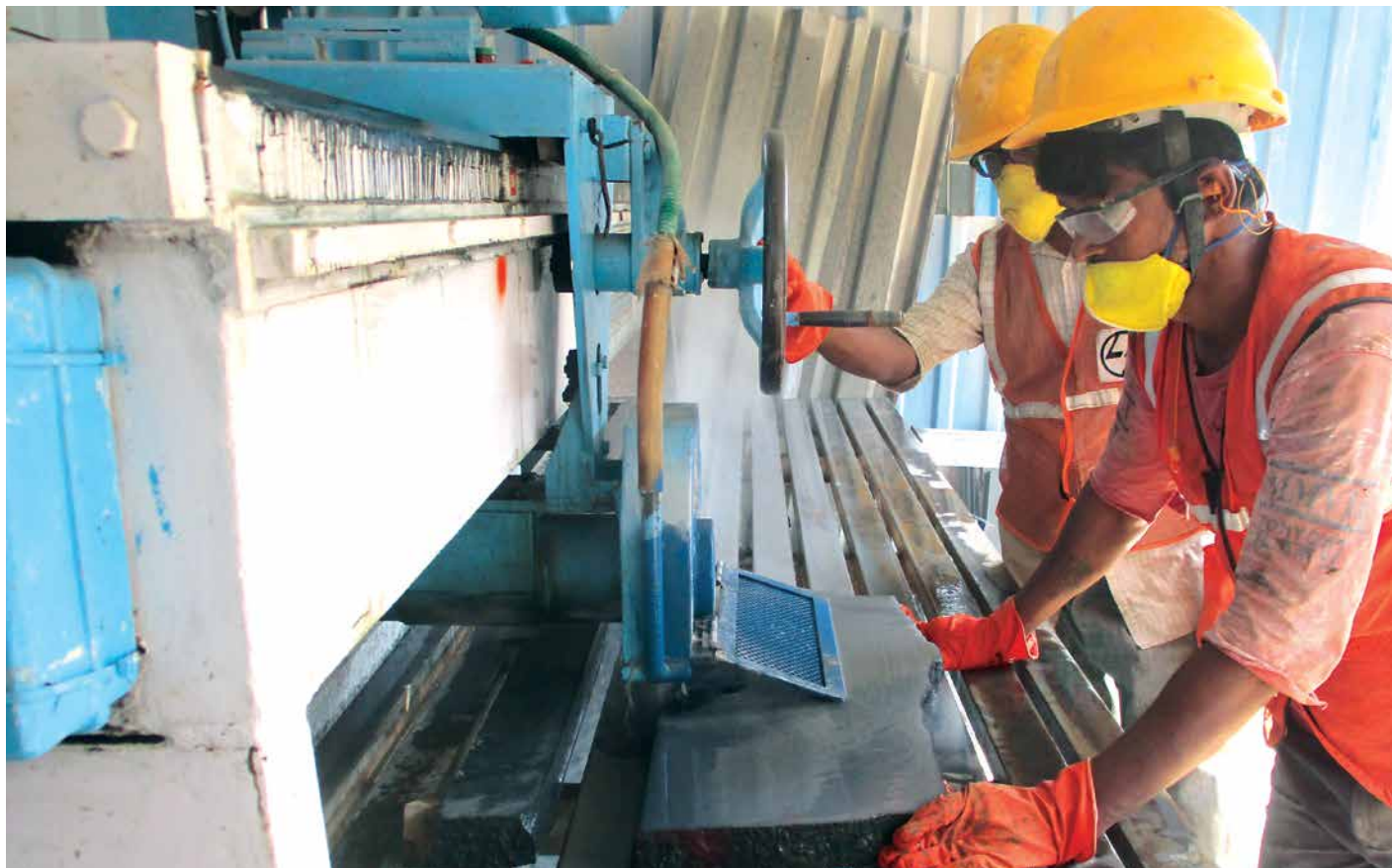
Closely inspecting finishing processes
