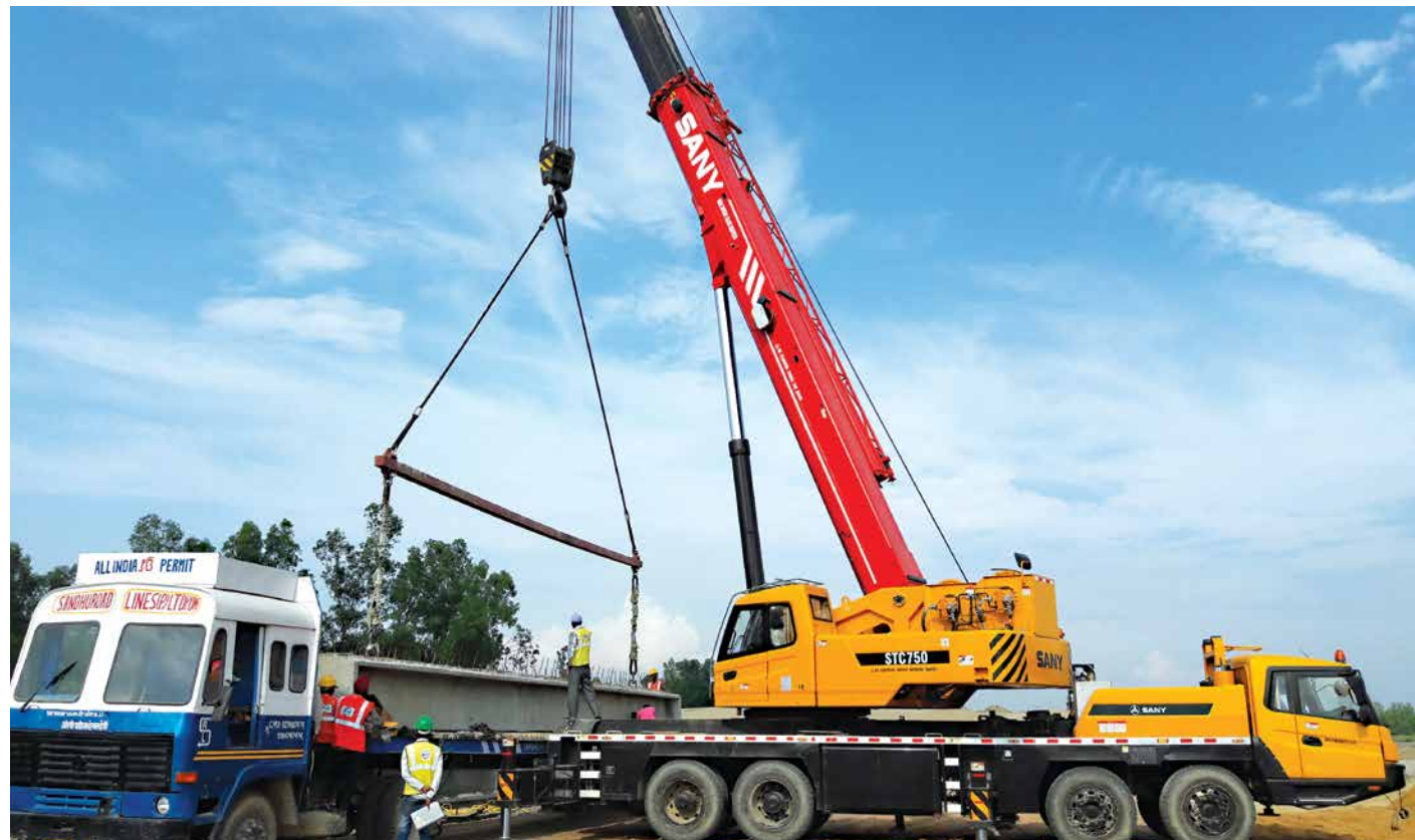
Lifting of precast elements
