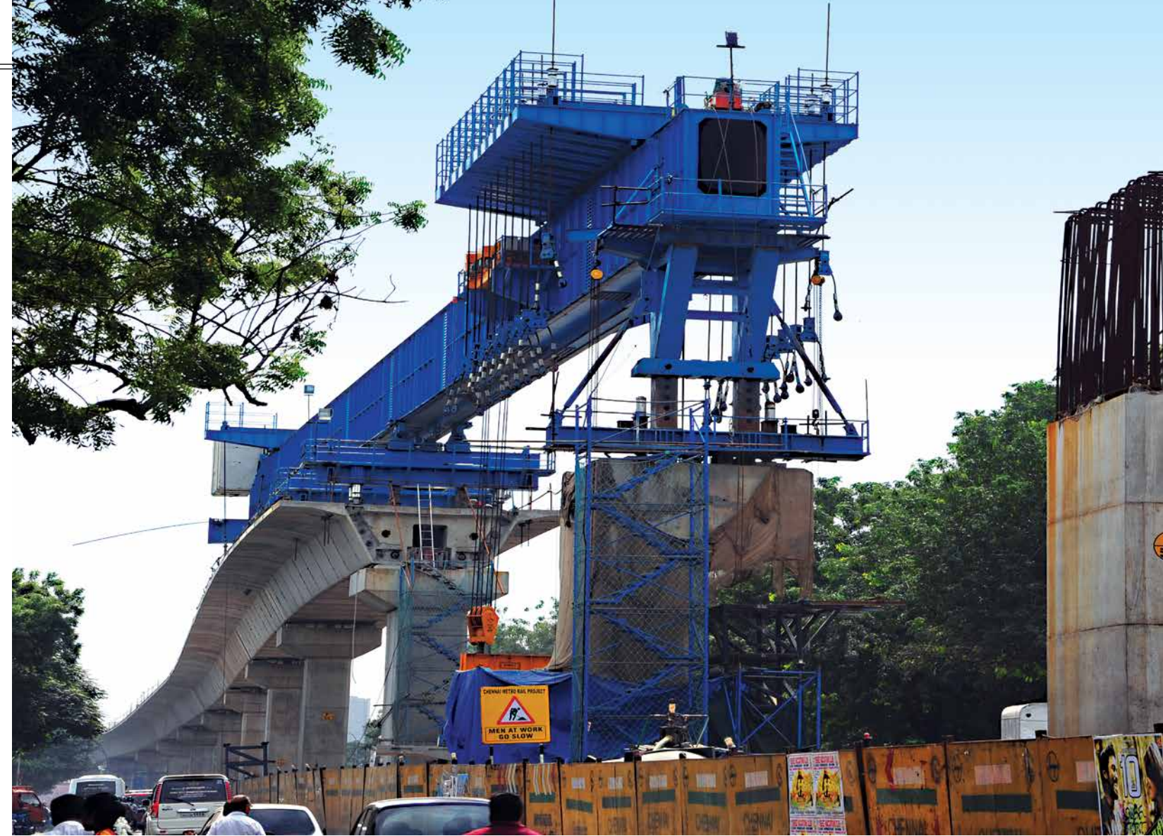
Girder erection across a busy junction
