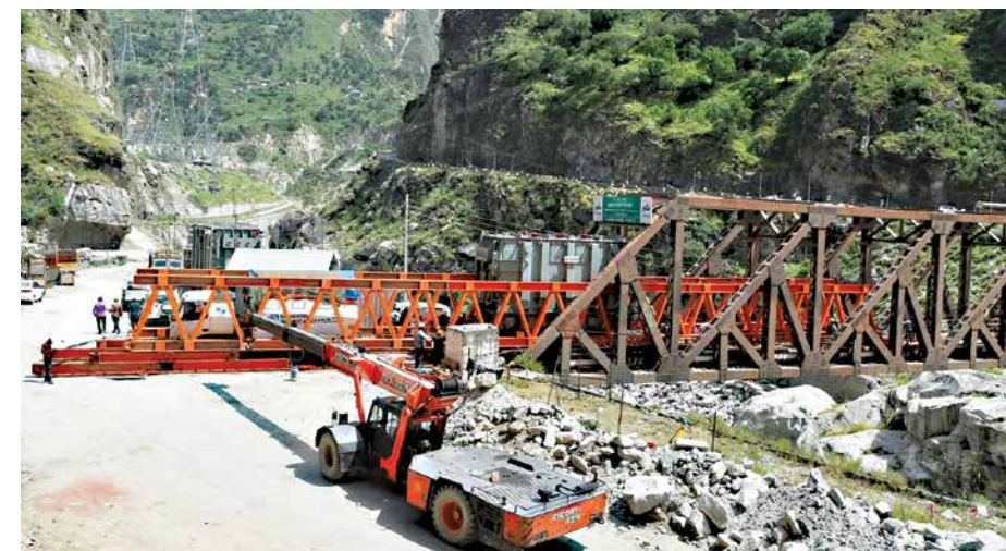
Configuring a safe method for moving a heavy weight transformer
