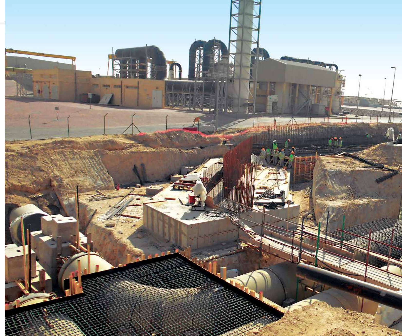
Deploying a safe zone work policy at the Jebel Ali STP
