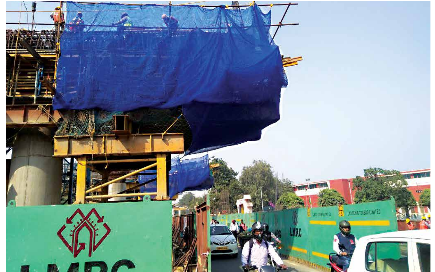
Providing complete cover with safety nets and barricading for an elevated metro corridor construction
