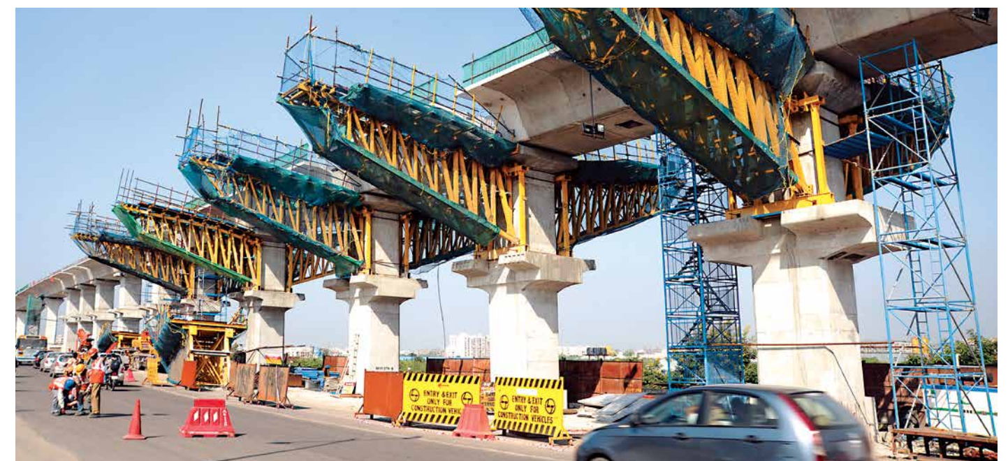
Safe barricading for an elevated metro rail corridor
