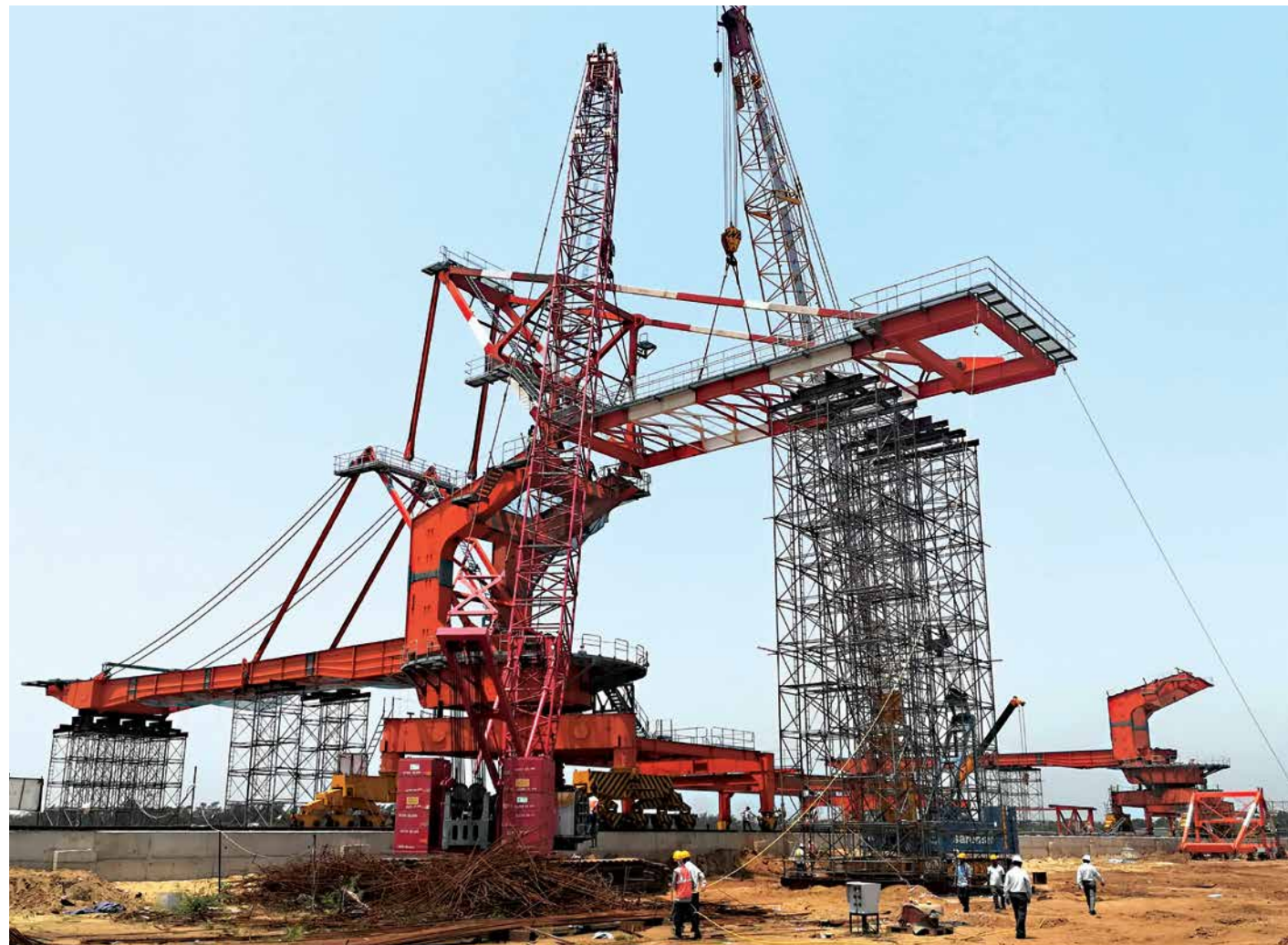
Erection of a stacker reclaimer at the Paradip Port Terminal
