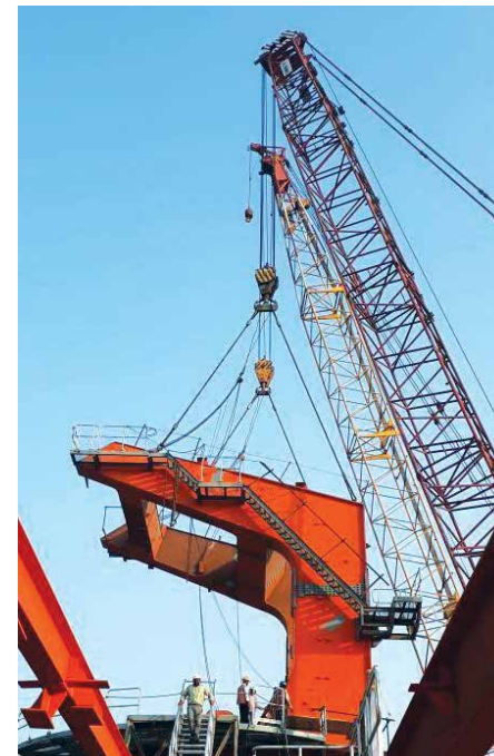
A complex lift in progress
