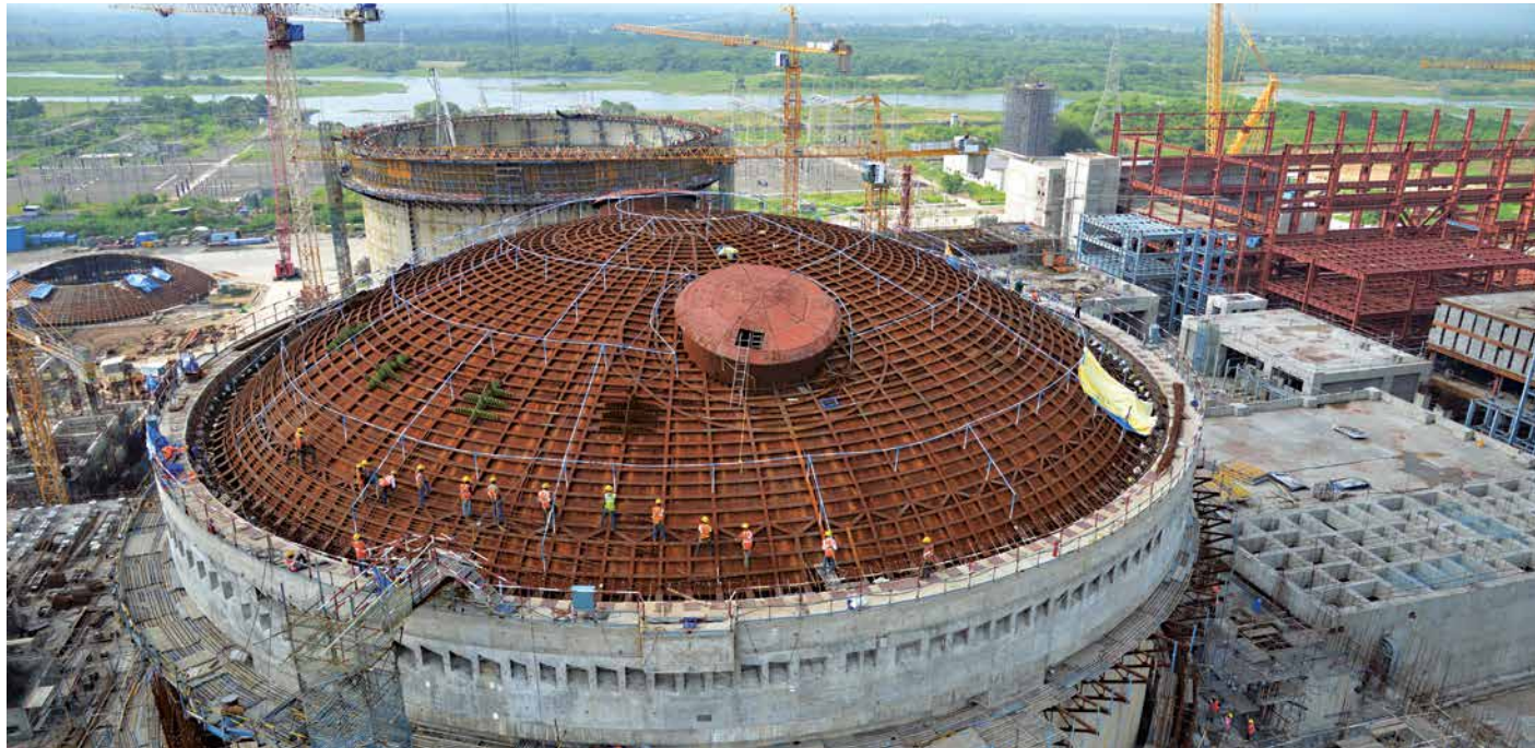
Workmen fixing the individual panels of the prefabricated ring liner at Kakrapar Atomic Power Project
