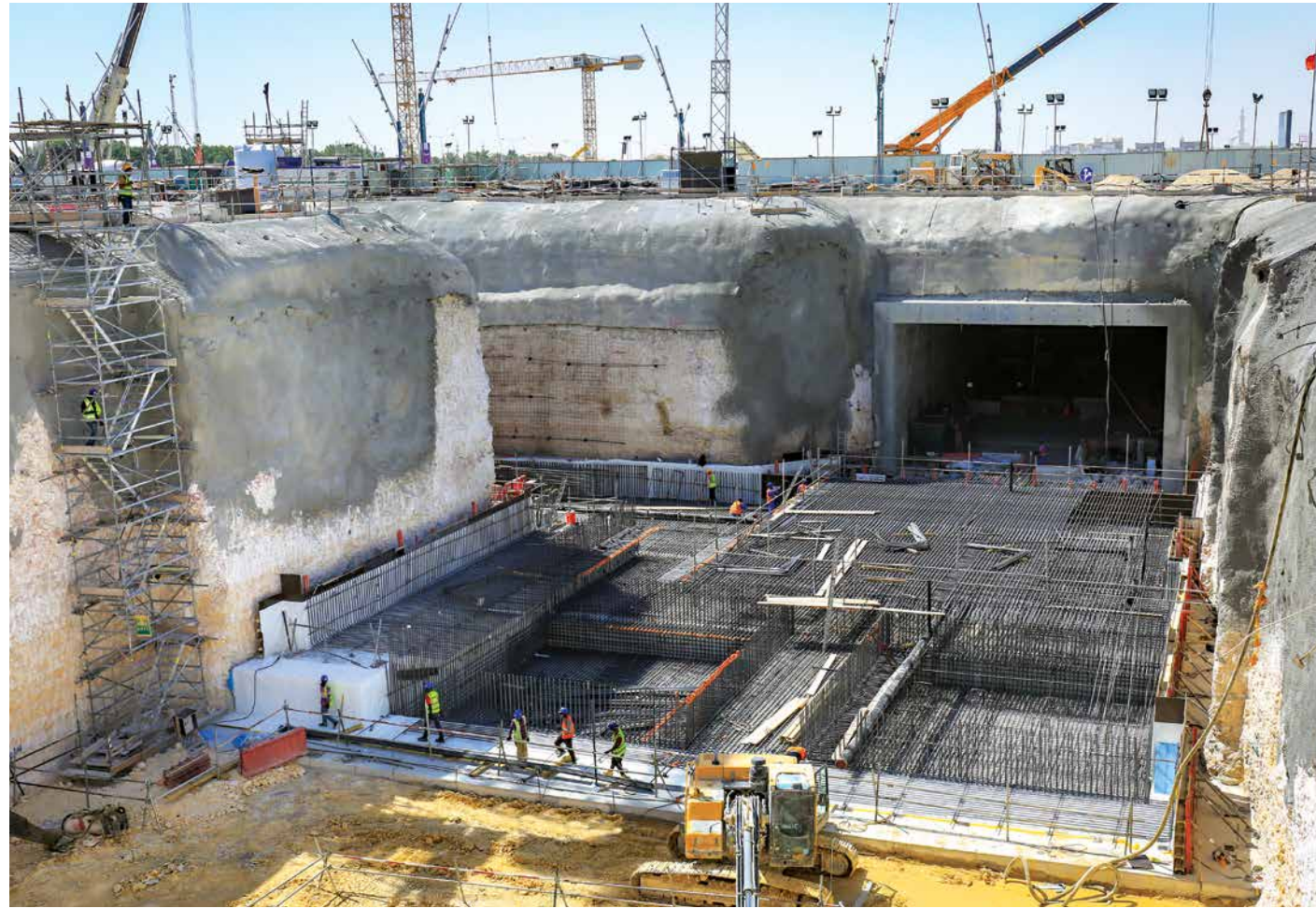
Base slab work in progress
