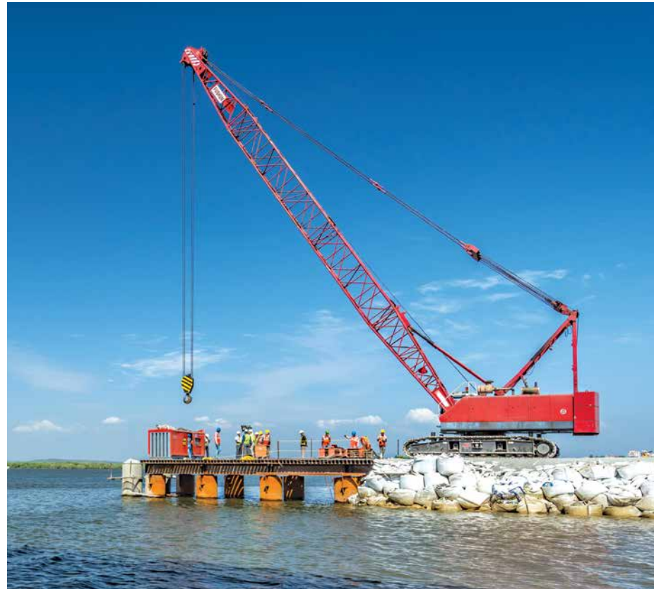
Safe placing of an equipment
