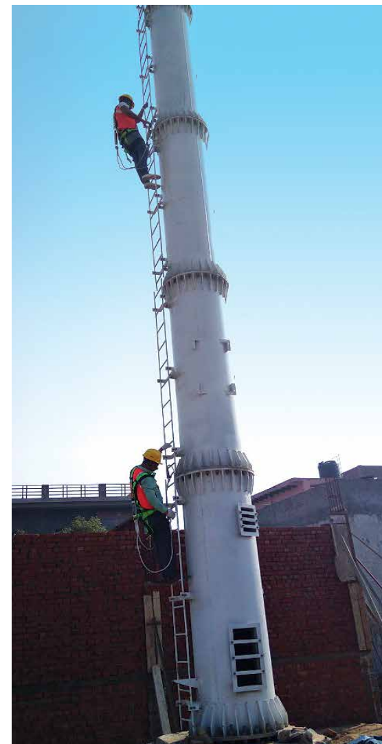
Climbing heights, hooked to life lines
