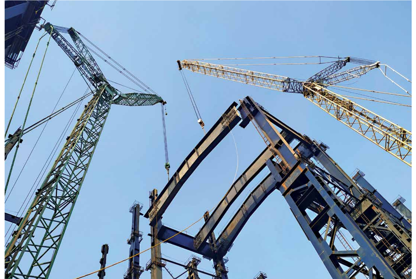
Rafter erection in high rise area at JSW Dolvi, SMS#2 project
