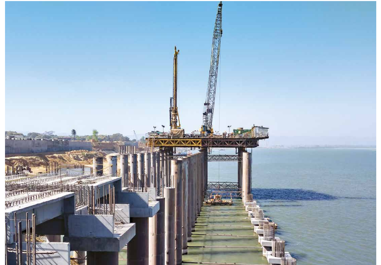
Multi-model terminal at Sahibganj, Jharkhand
