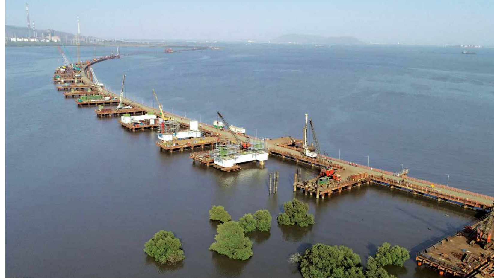
Bridging the sea at the Mumbai Trans-Harbour Link project
