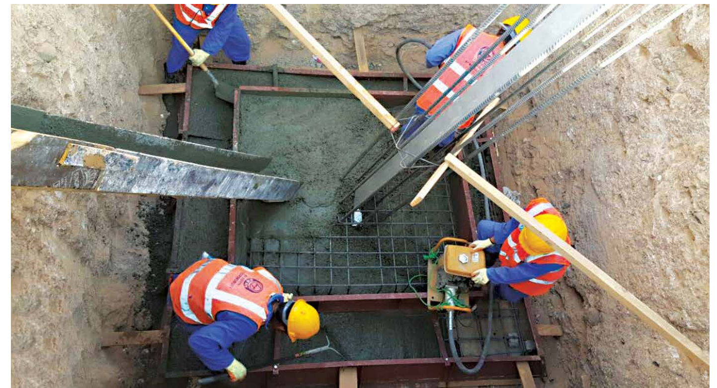
Establishing firm footings
