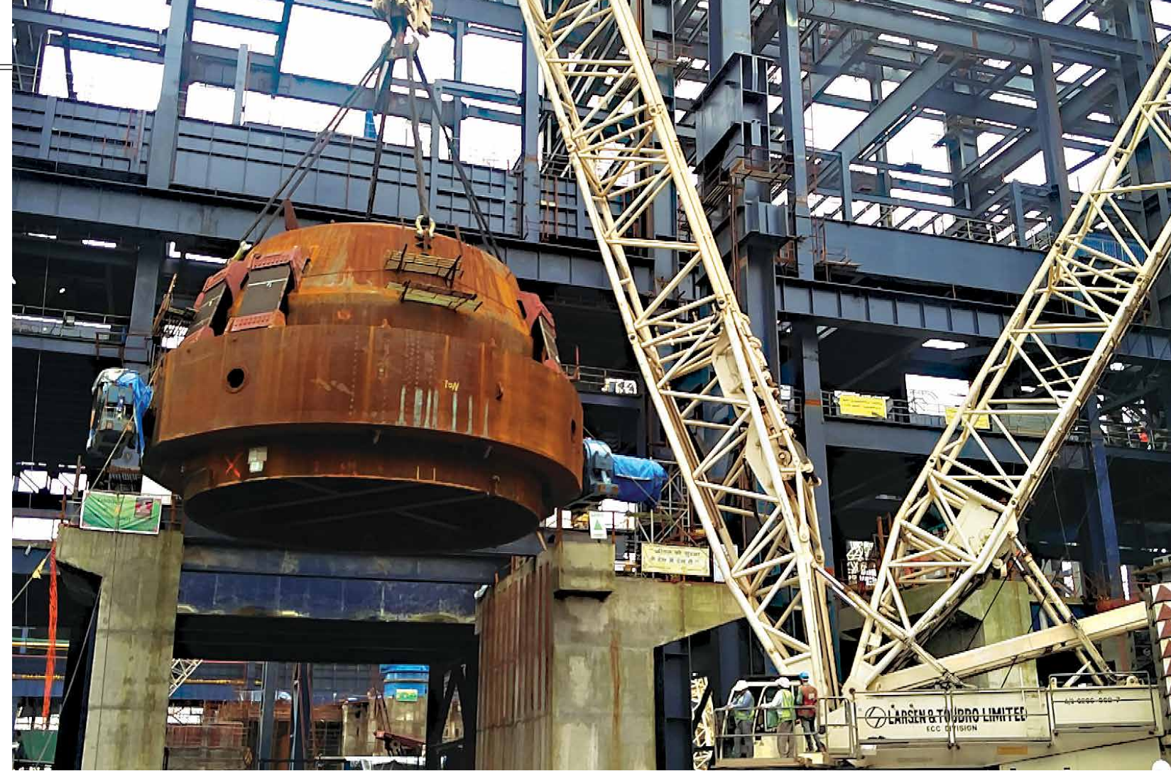
Erection of converter at JSW Dolvi, SMS#2
