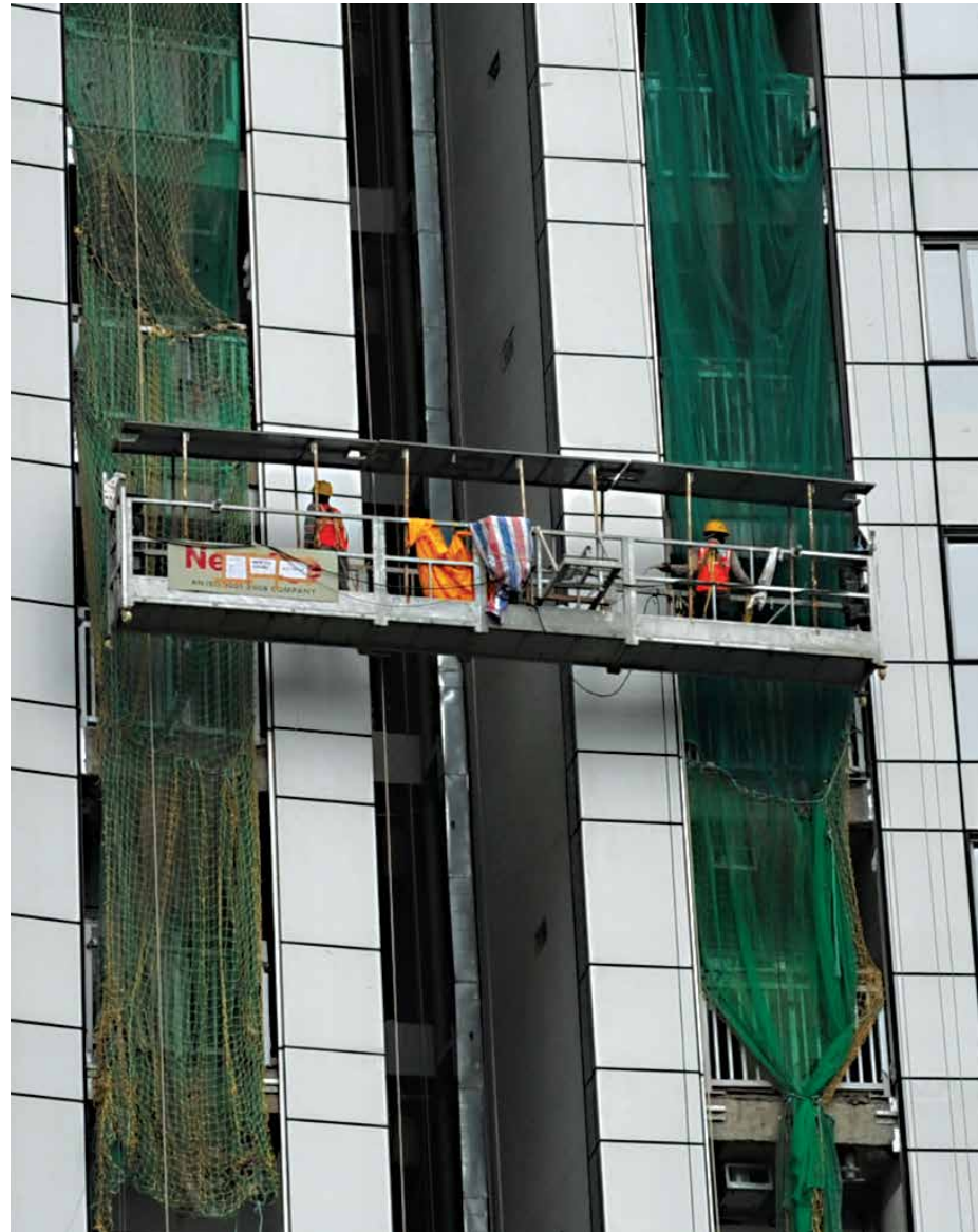
Accessing heights with a safety climbing screen
