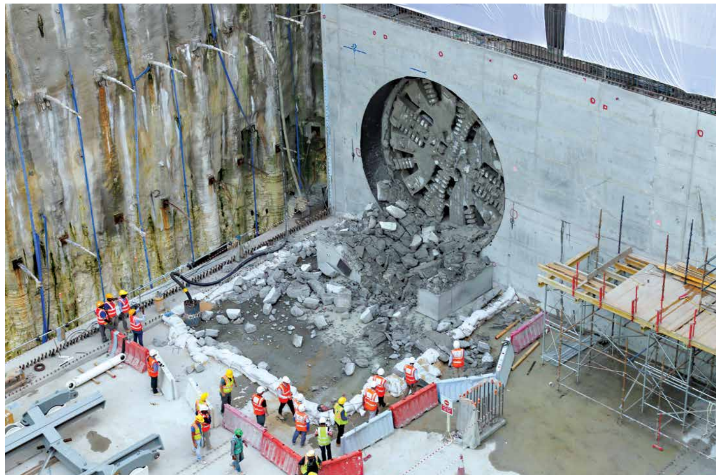
TBM (Tunnel Boring Machine) in action at Riyadh
