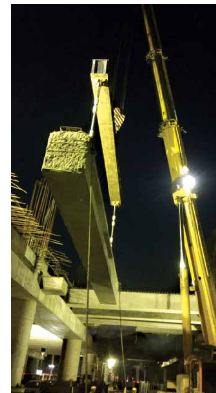
Lifting of girders in the middle of the night
