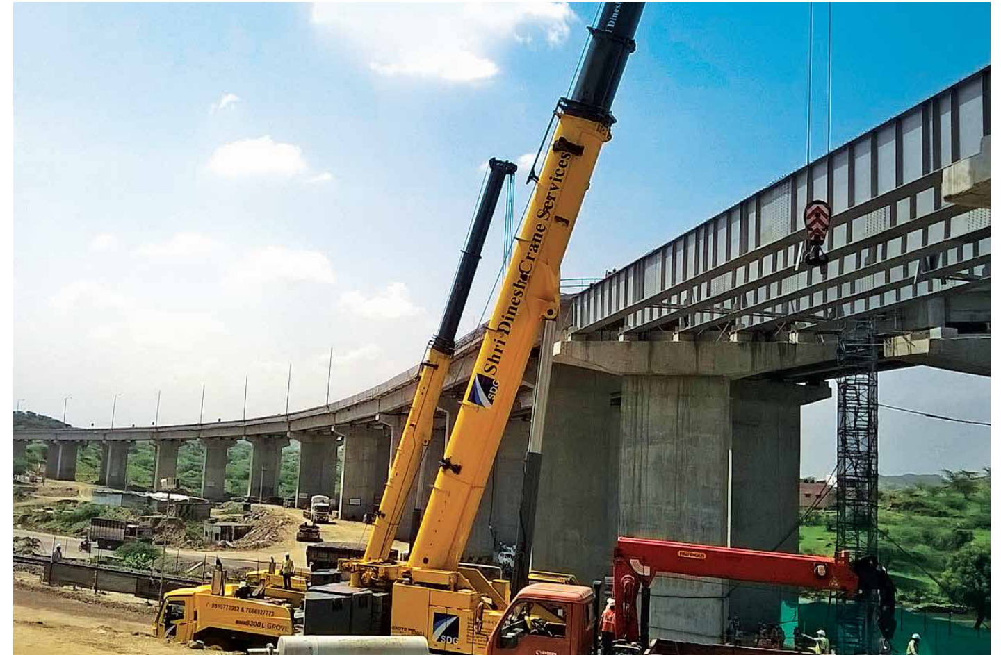
A critical steel girder erection
