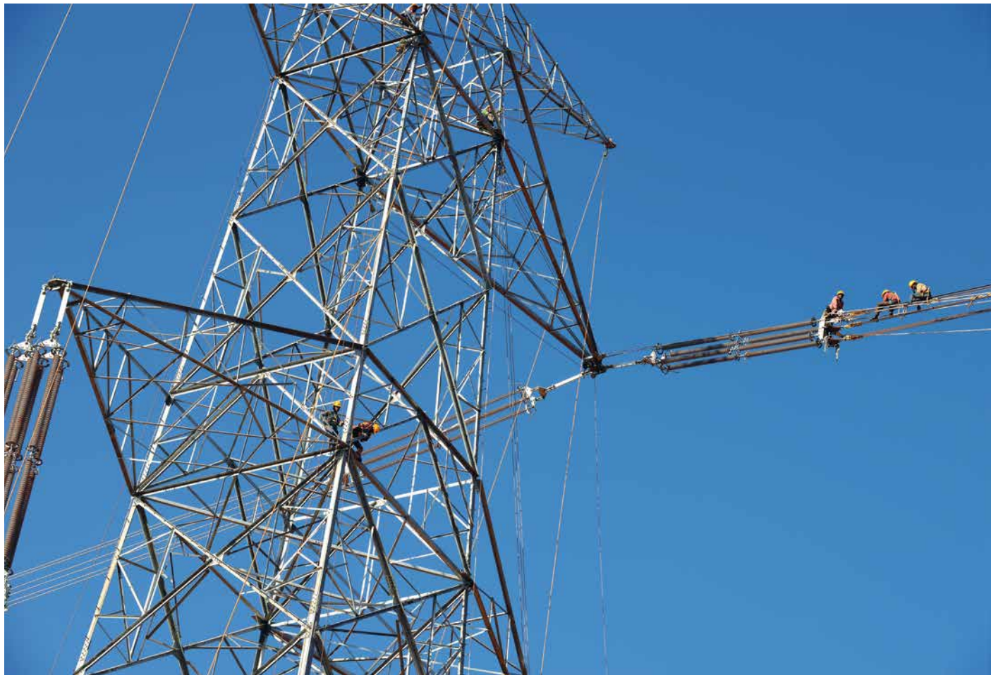
Workmen on lifelines to raise the steely tower members
