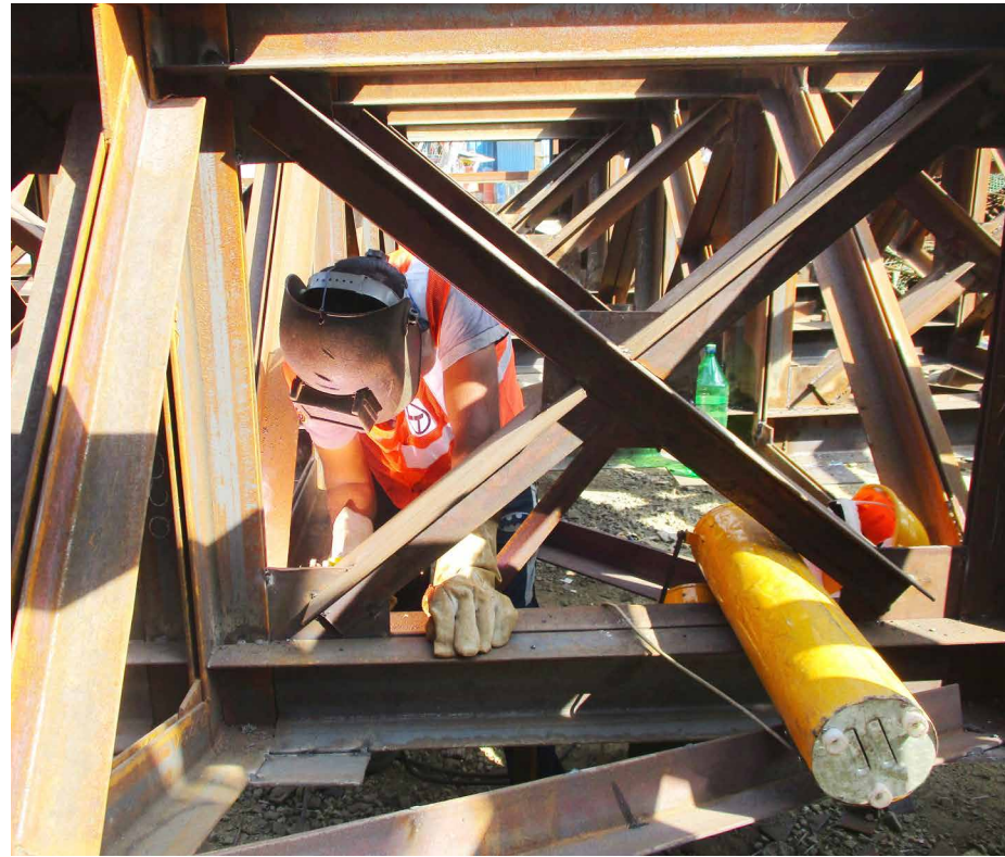
Fabrication works for entrance portal
