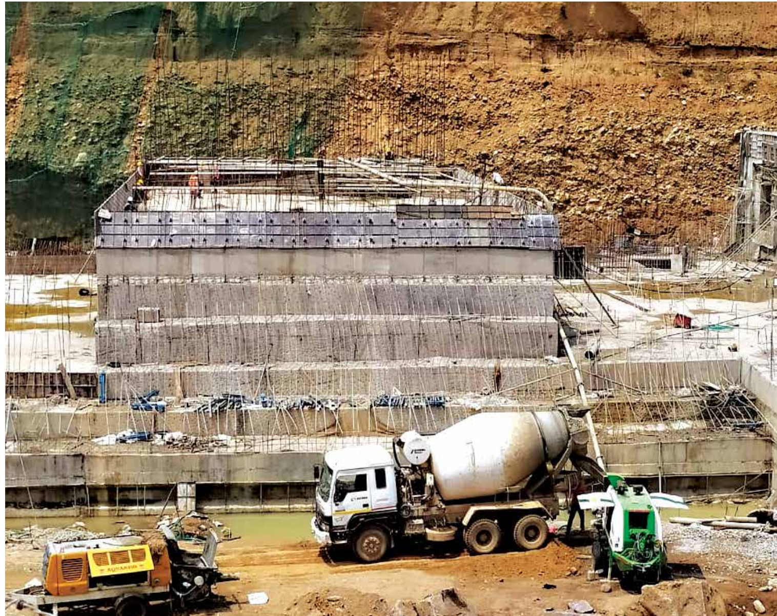
Concrete of 720 Cum poured at Runj Dam project in Panna (Madhya Pradesh)
