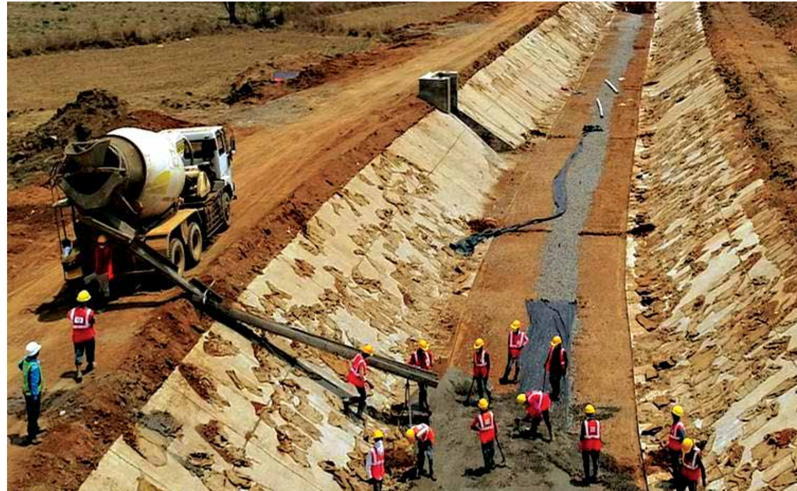
Canal bed concreting
