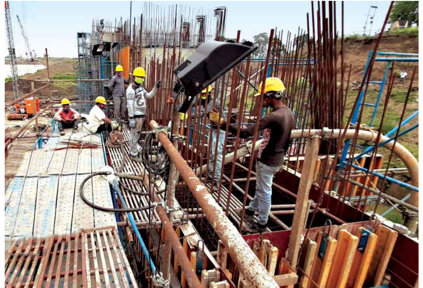
Concreting work for Critical Counterfort wall, with a pour of 7 m length, second lift for 36 Cum at the Farakka site
