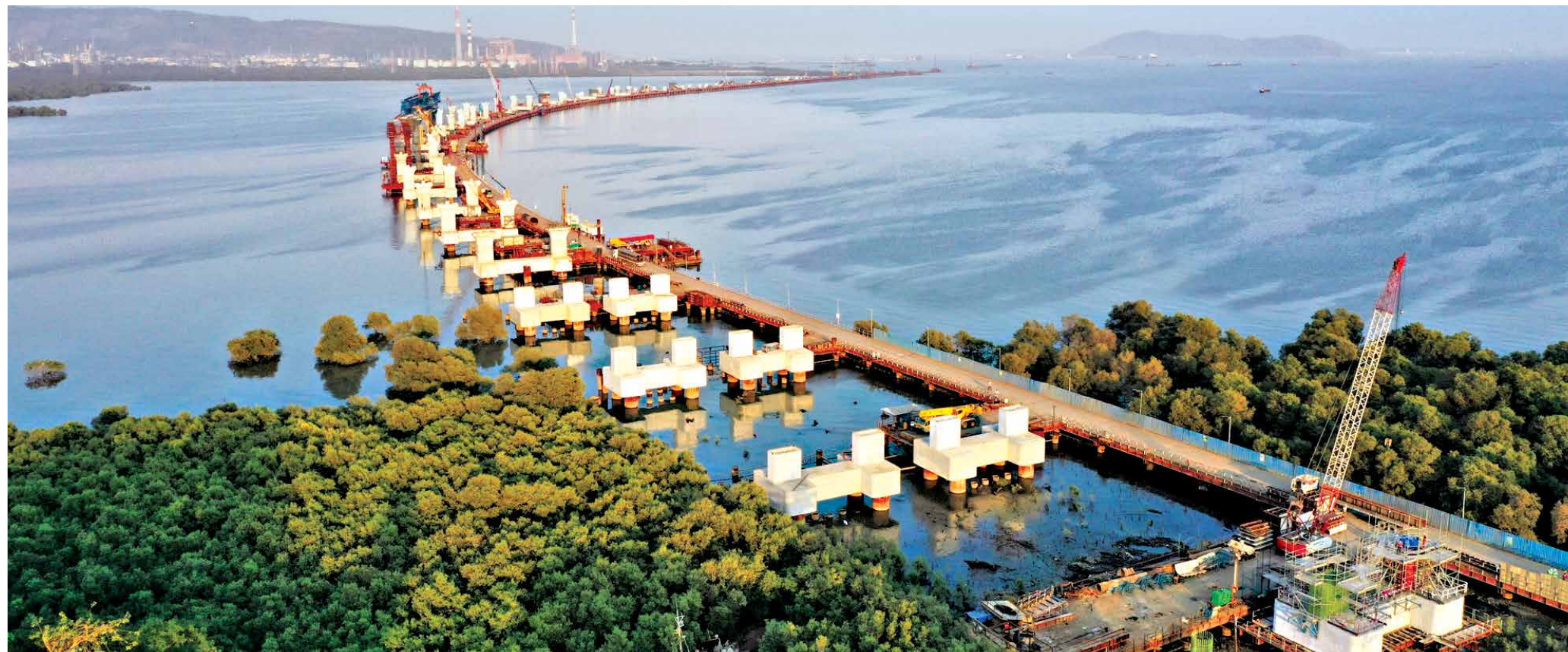
Mumbai Trans Harbour Link Project
