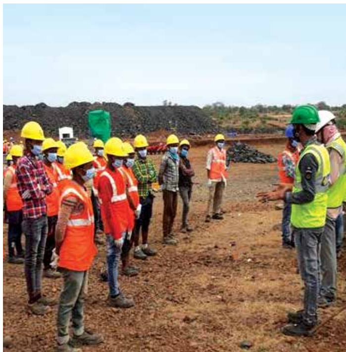
SOPs being briefed to workmen
