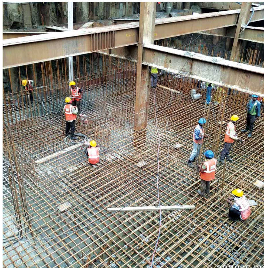
330 Cum of concrete up to 16 m below ground level poured in one day at JSW Paradip site
