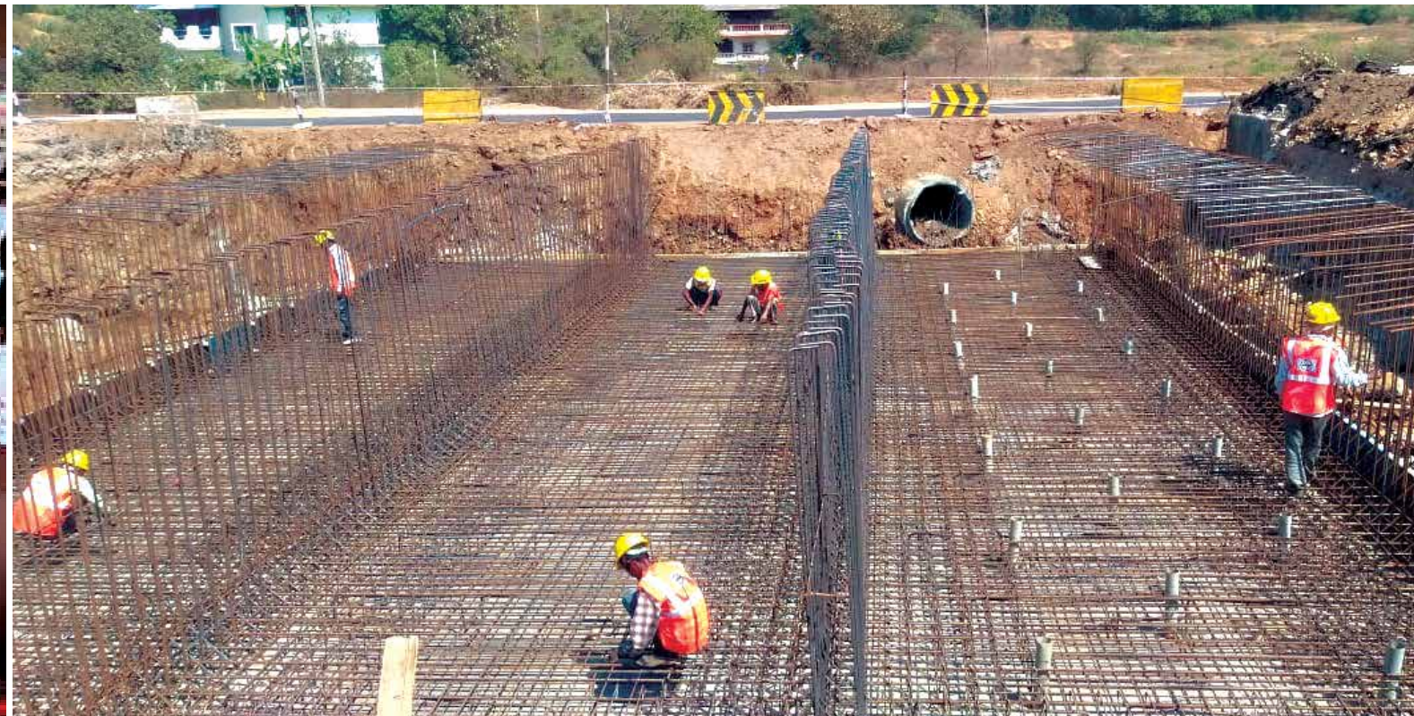
Workmen involved in rebar works maintaining social distancing
