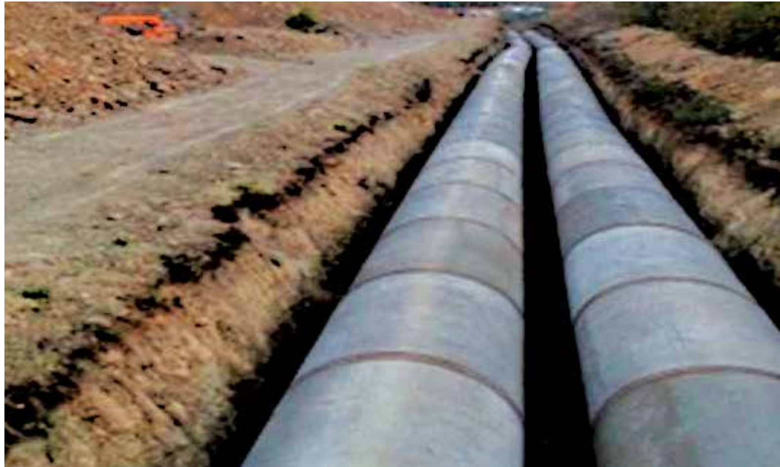
Laying of 3110 mm dia twin pipeline
