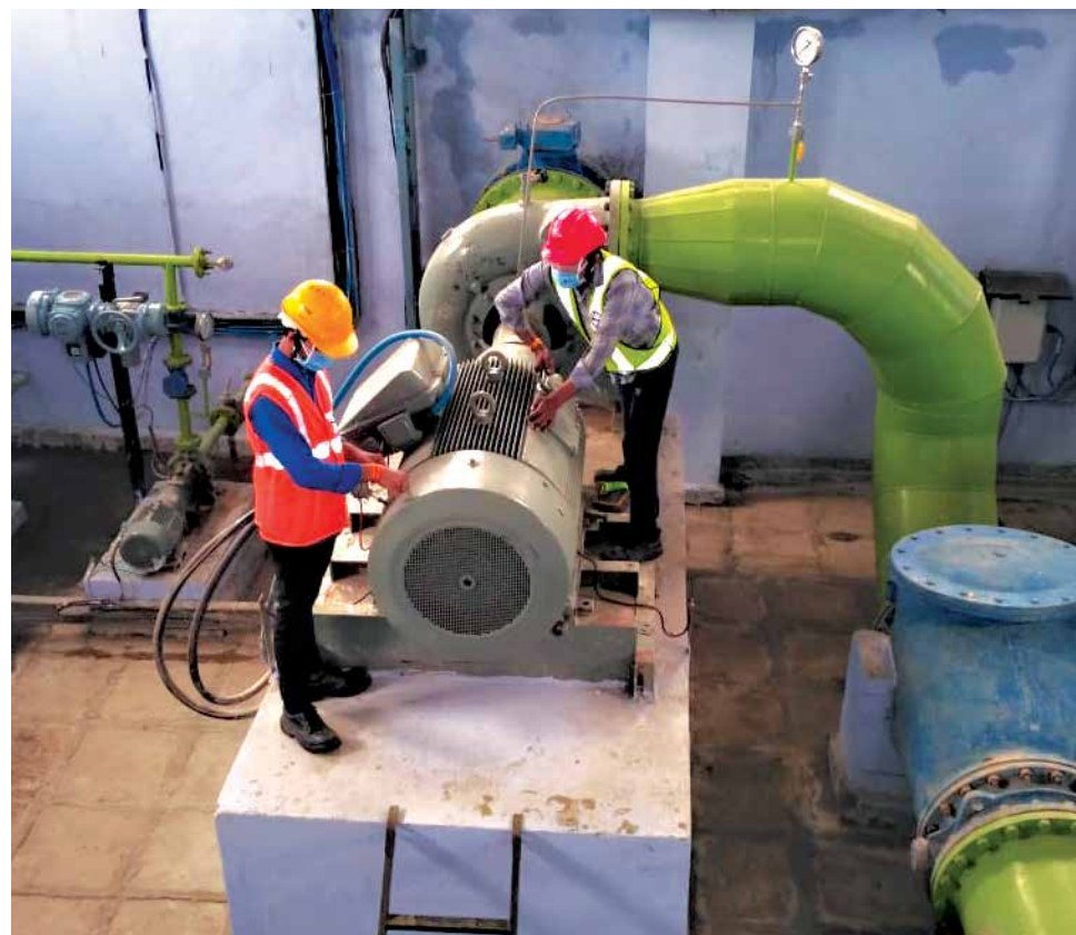
Pump maintenance at the Pithampur Industrial Water Supply Plant
