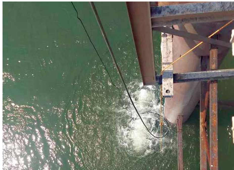
Contained air bubbles generated out of controlled vibration during piling operation
