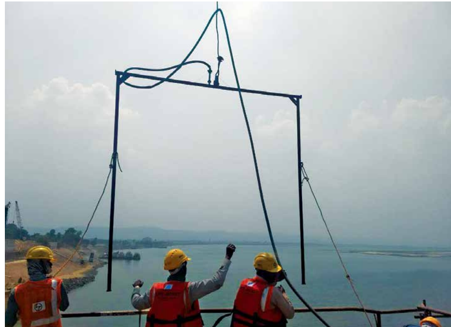
Air bubble curtain set up being lowered close to pile location
