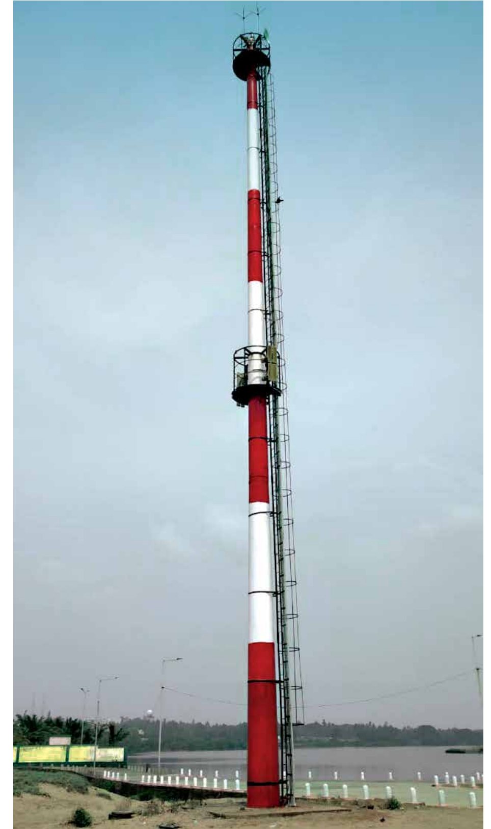
30 meter spun concrete tower for Alert Siren System
