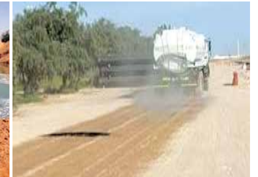
Re-use of water for dust suppression
