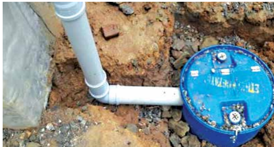
Rainwater harvesting pits
