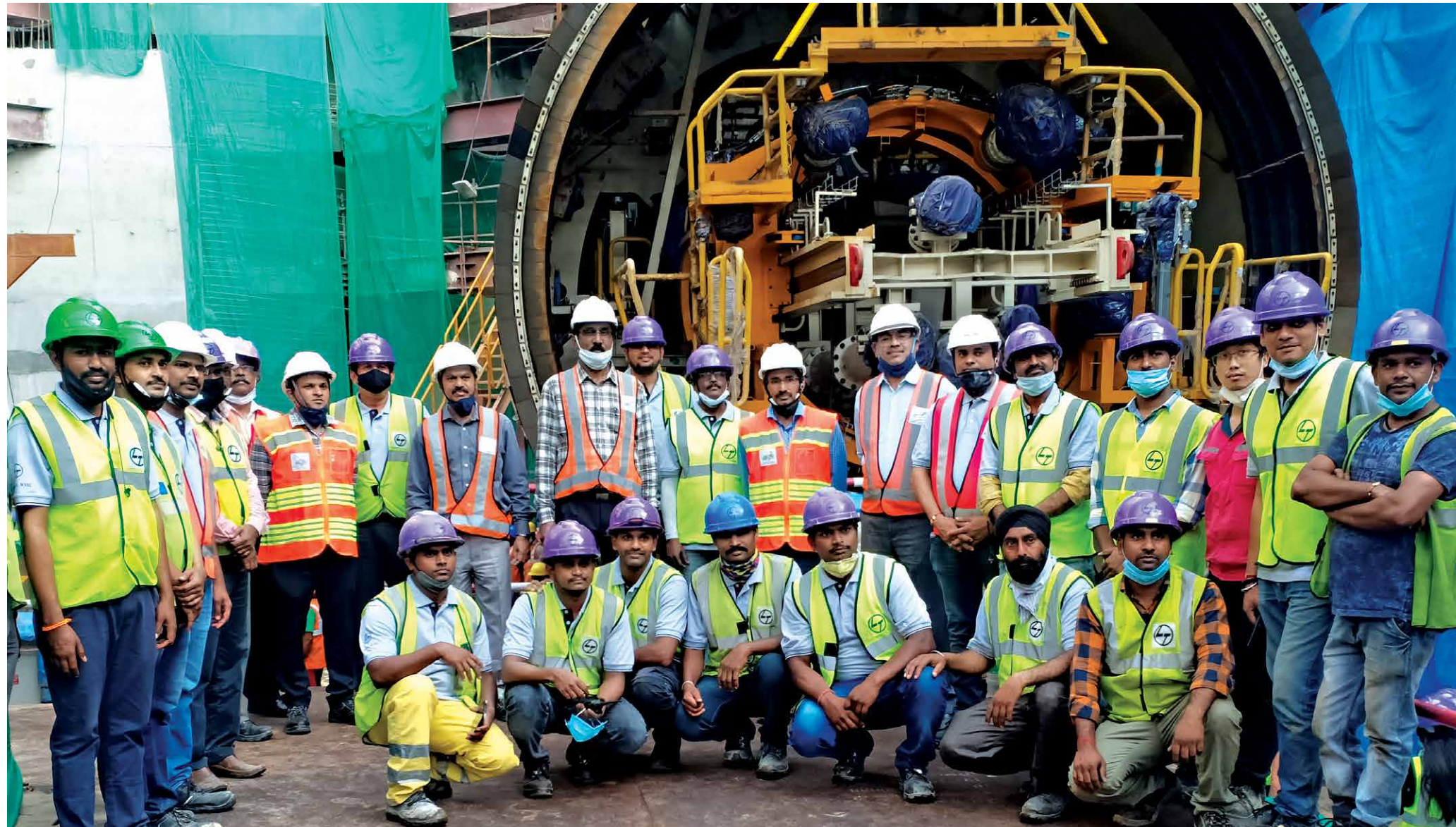
Launch of TBM Avni at BMRL RT 02
