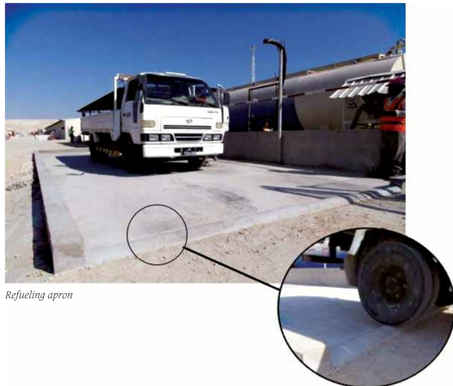
Secondary containment for prevention of fuel spillage
