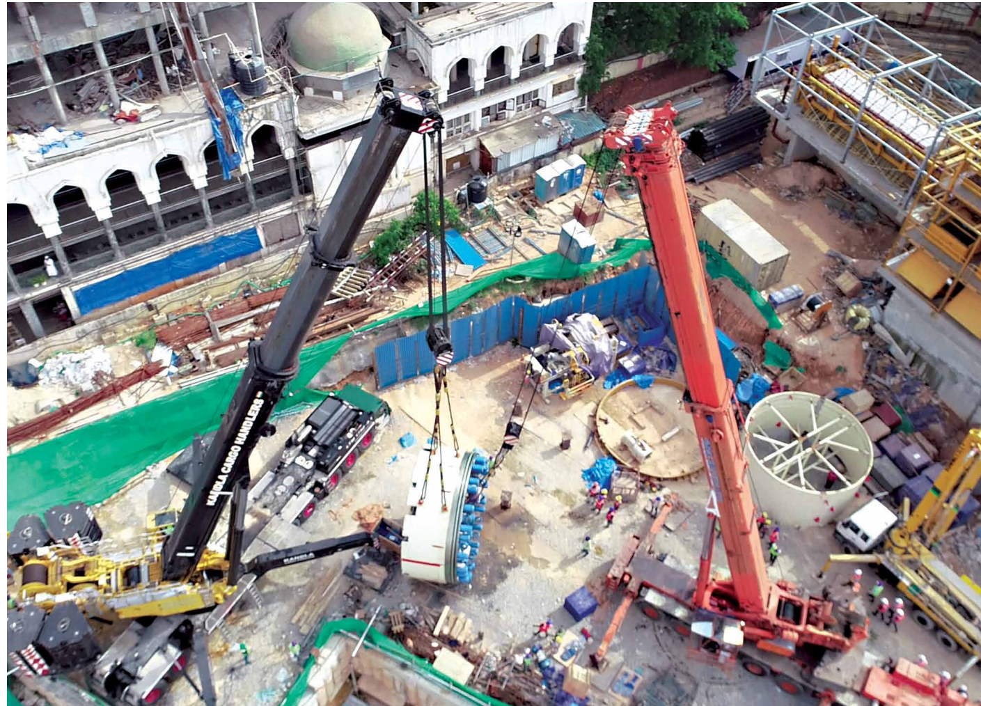
TBM 1 (AVNI) auxillary shield tandem lifting & lowering in progress
