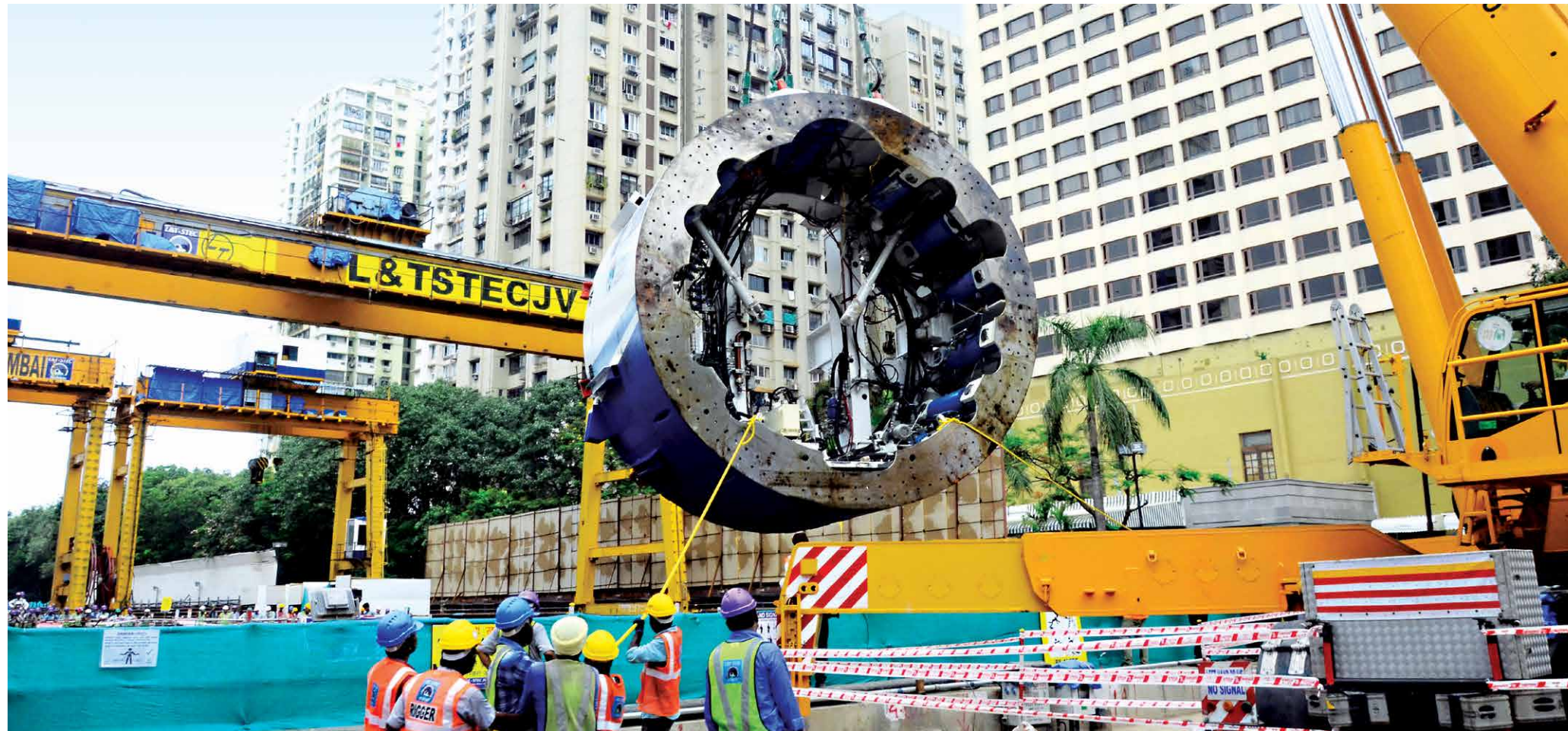
TBM shield being lifted at Mumbai Metro Package 03 UG 01
