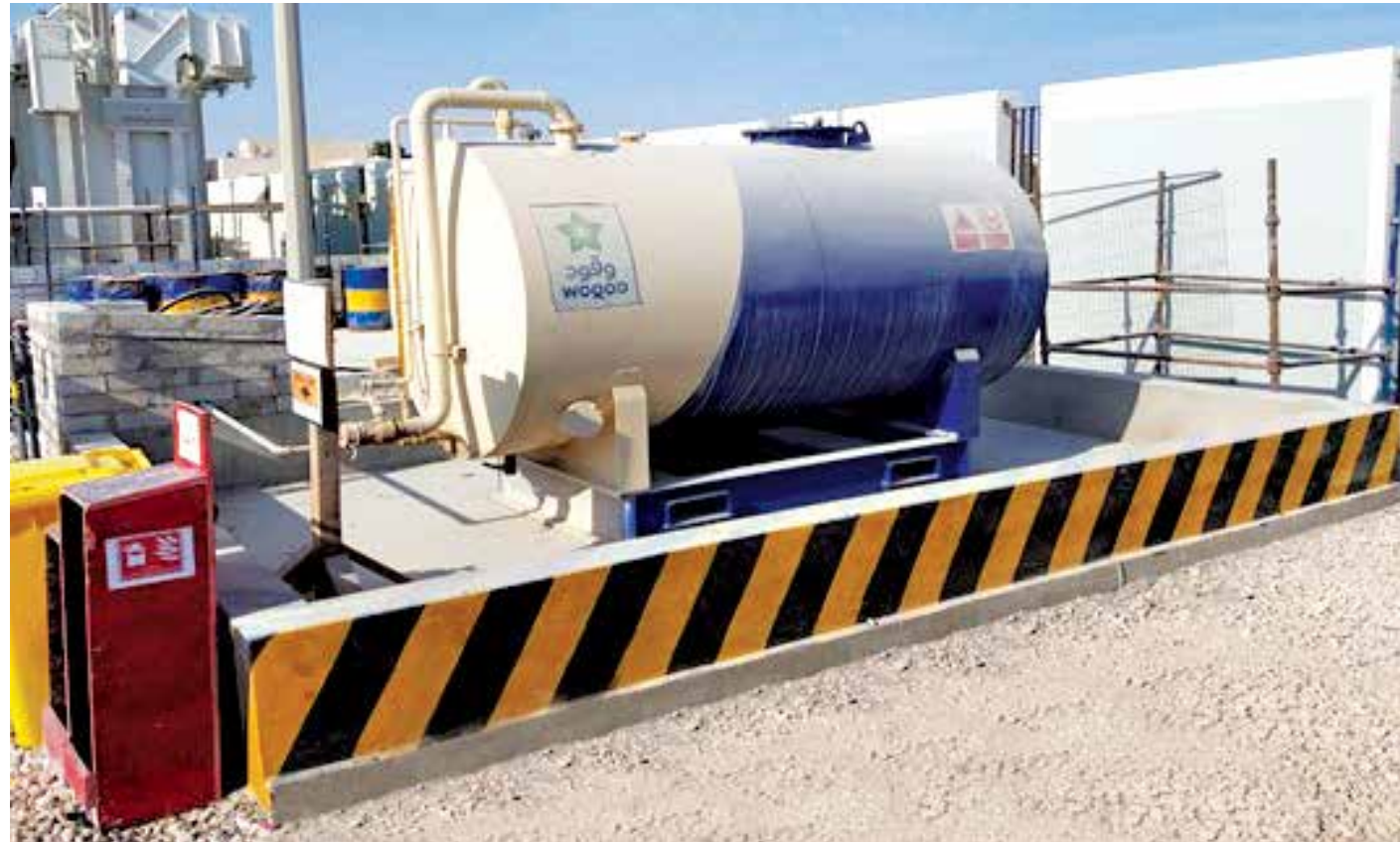
Secondary containment for prevention of fuel spillage
