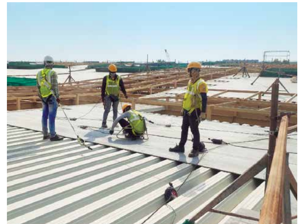
Roof work - Fall restraint systems
