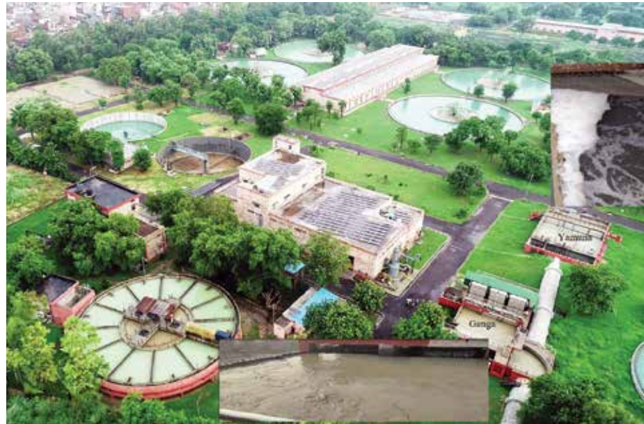
Overview of the plant with the Ganga and Yamuna inlet channels
