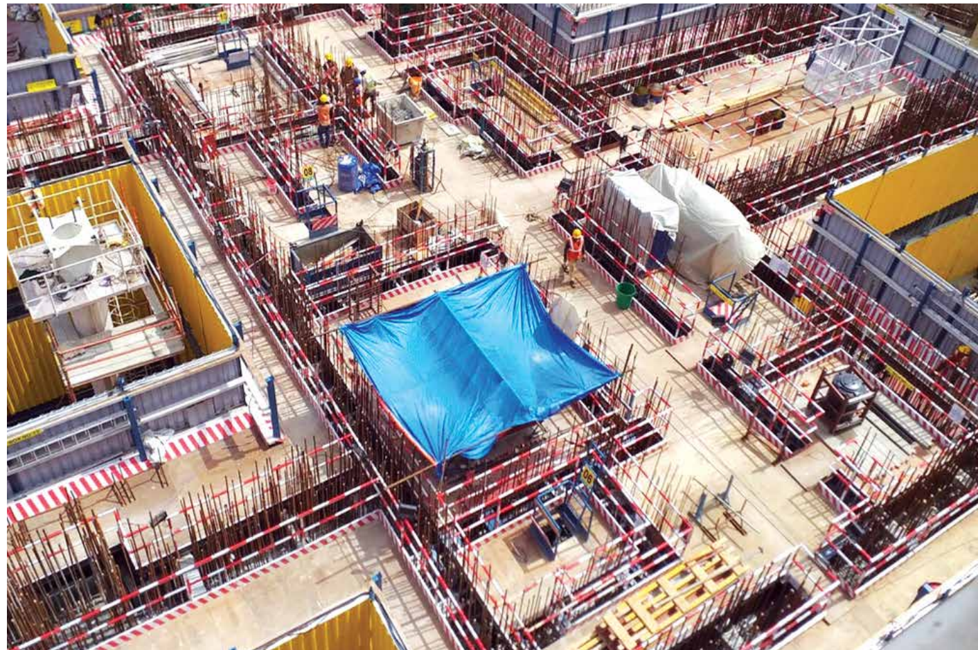
Aerial view of the Autoclimbing Formwork System
